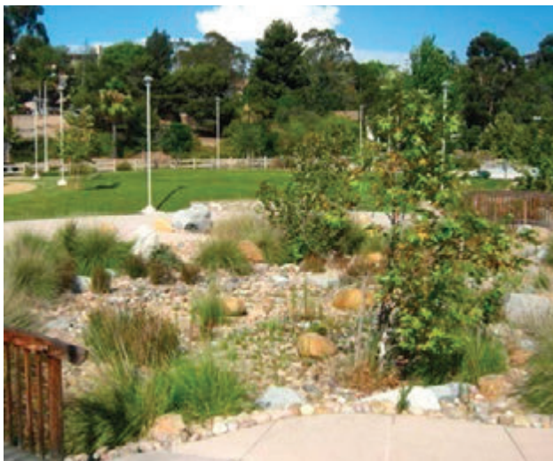
Planted bioswale with boulders
