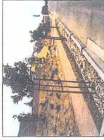
This schematic shows the major components of a rock infiltration swale. The rock infiltration swale in the photograph intercepts roadway runoff through curb cuts and filters it through subsoil water table.
