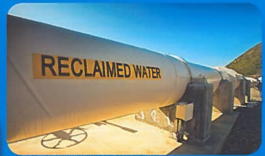
24-inch recycled water pipeline
