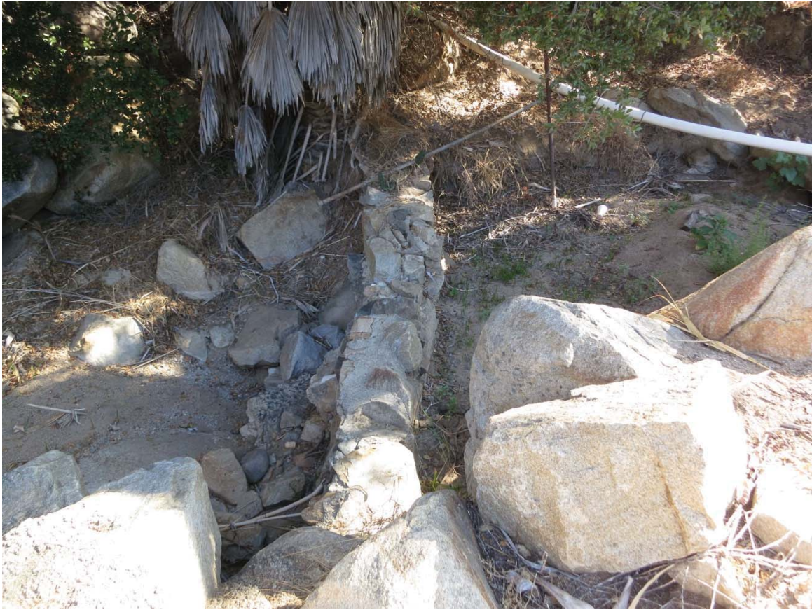
Figure 7. Grouted Riprap Check Dam near Lower End of Reach 2
