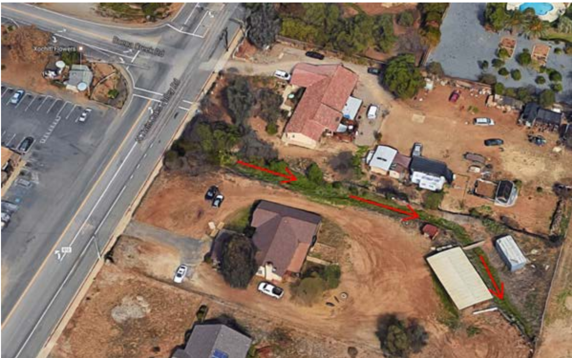
Basin 2000 Outlet – Downstream open channel
