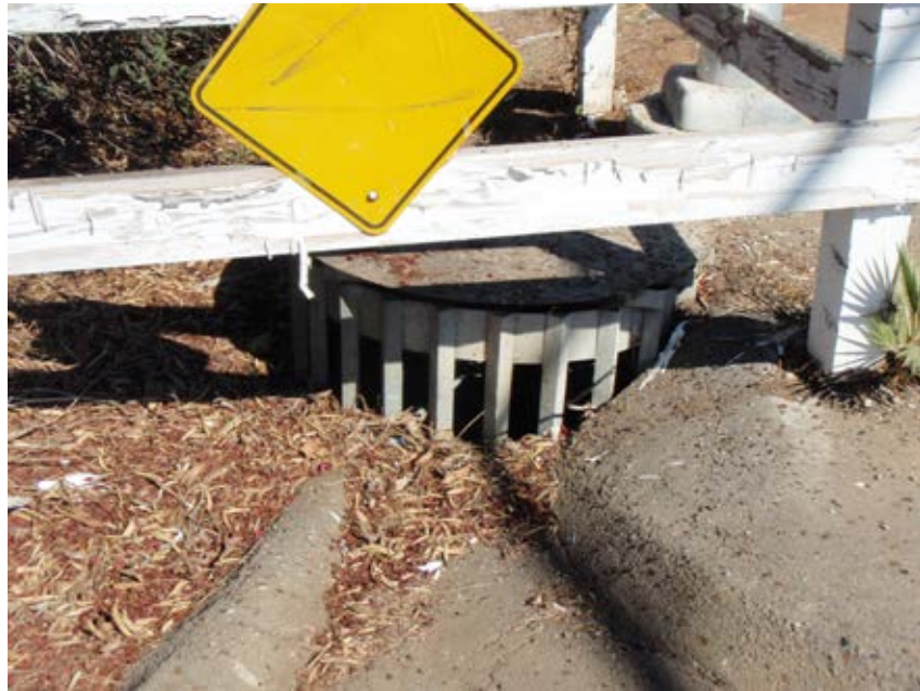
Basin 6000 Inlet – NW Corner Cassou Road
