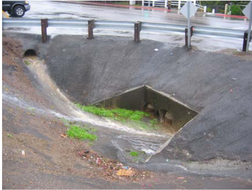
Basin 2000 Inlet – SW Corner Buena Creek Road
