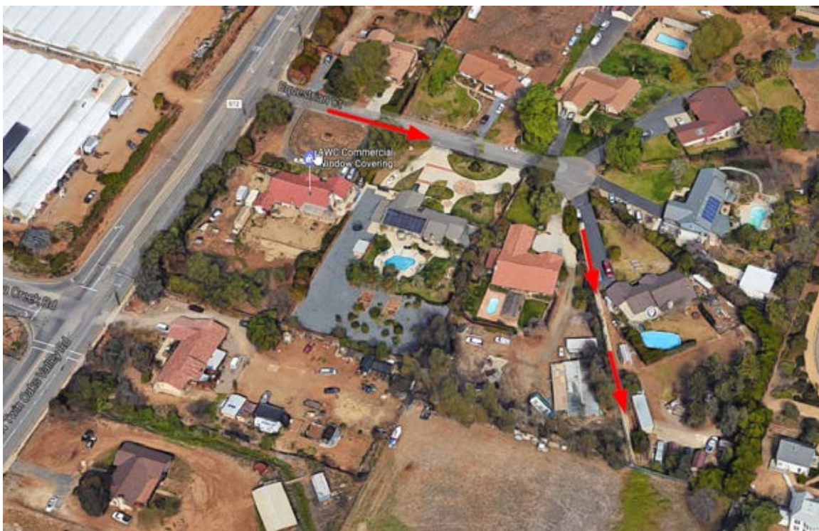
Basin 4000 – Downstream to concrete swale/open channel
