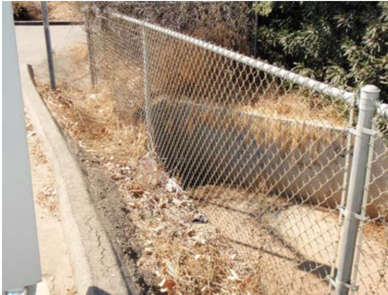
Basin 1 Inlet – West Side Twin Oaks Valley Road
