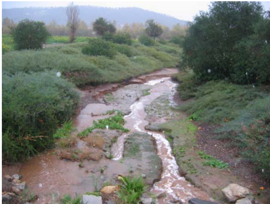
Basin 1 Outlet – Downstream Open Channel
