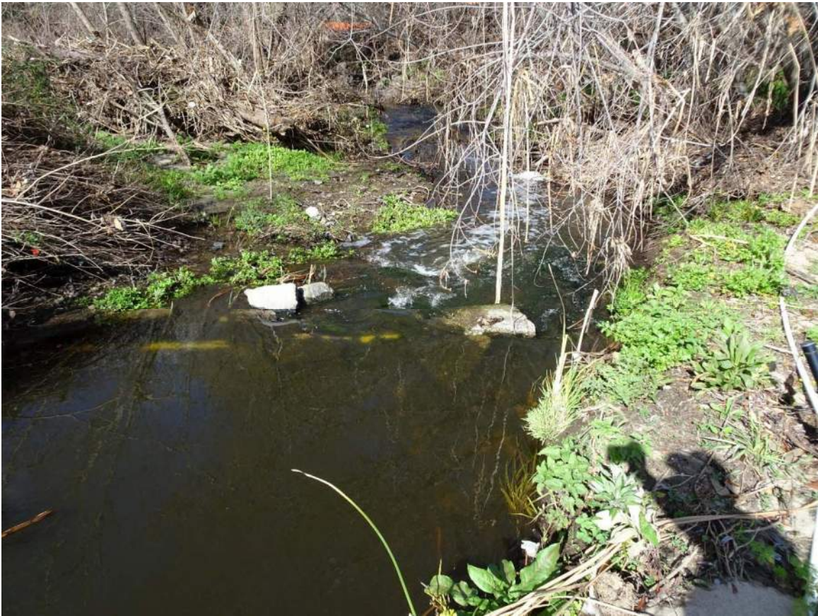
Figure 5. Concrete Grade Control between Reach 1 and Reach 2
