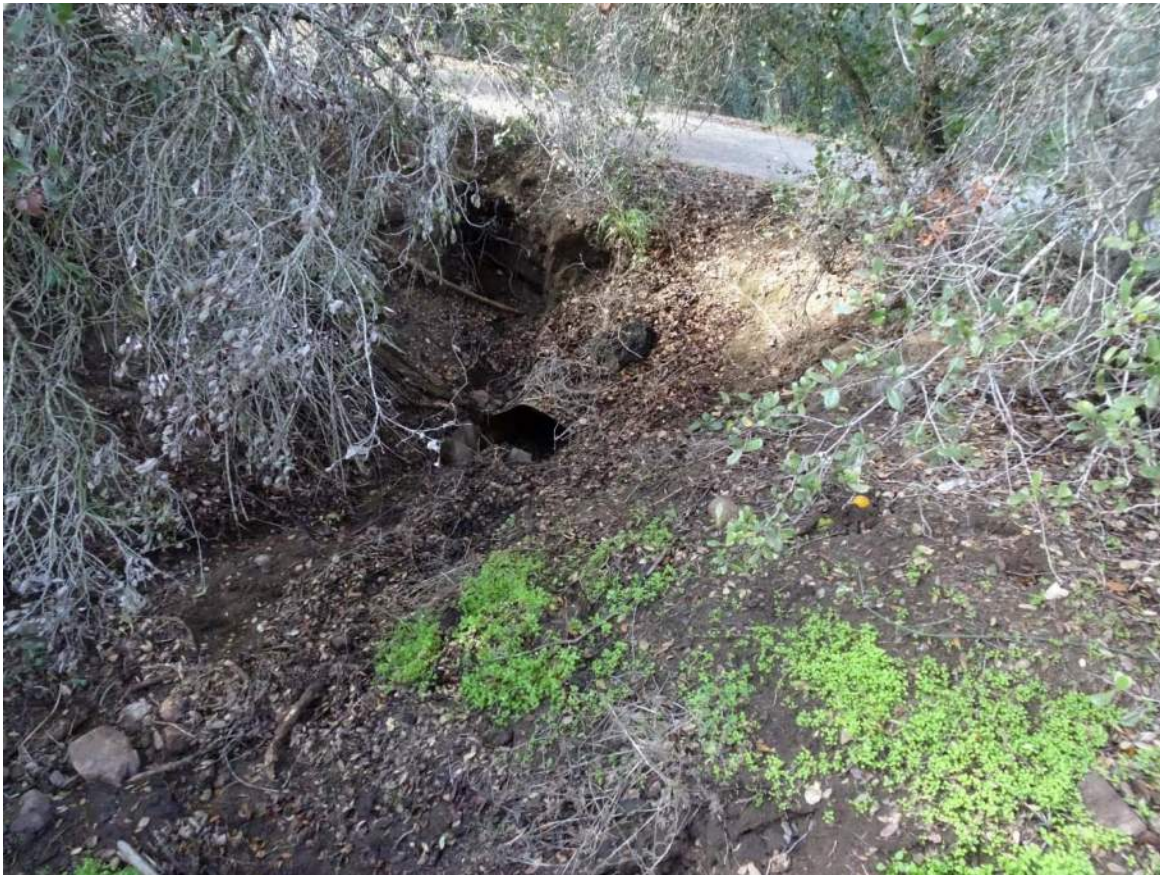
Figure 11. Culvert (Grade Control) under Cordrey Drive at Downstream End of Reach 4
