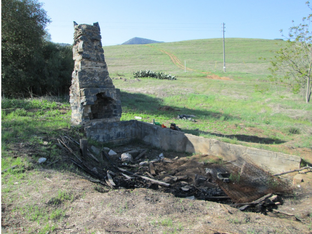
Figure 4. Southwest view of main complex from northeast corner of the front porch.
