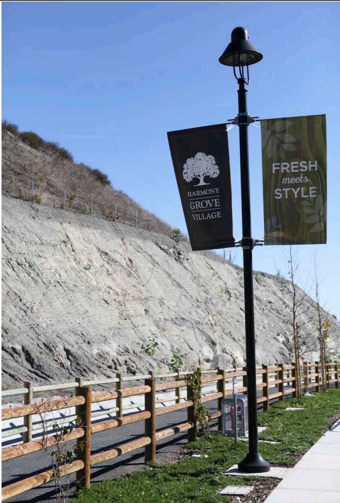
HGV Sidewalk, Pathway and Slope Adjacent to Roadway
