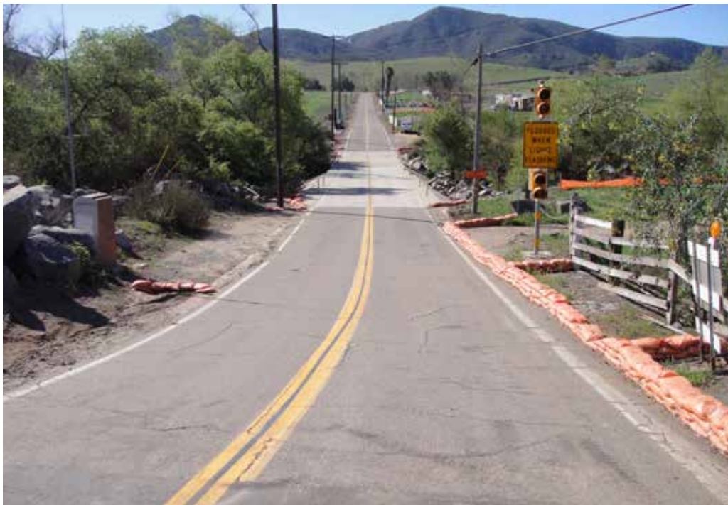
Photo 1: View of existing low-water crossing for Country Club Drive over Escondido Creek in northern portion of the study area, facing south. A new bridge is proposed at this location that will remove the existing low-water crossing, improve wildlife movement functions, and restore riverine hydrology.
