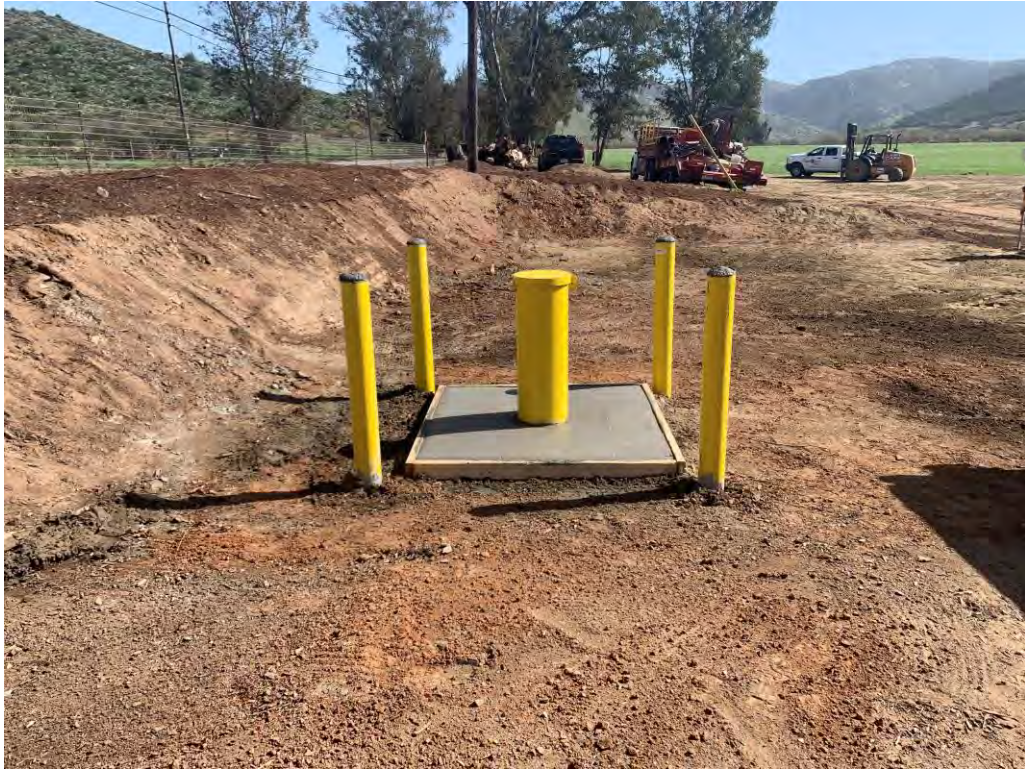
Photograph 9 - SP129 surface completion
