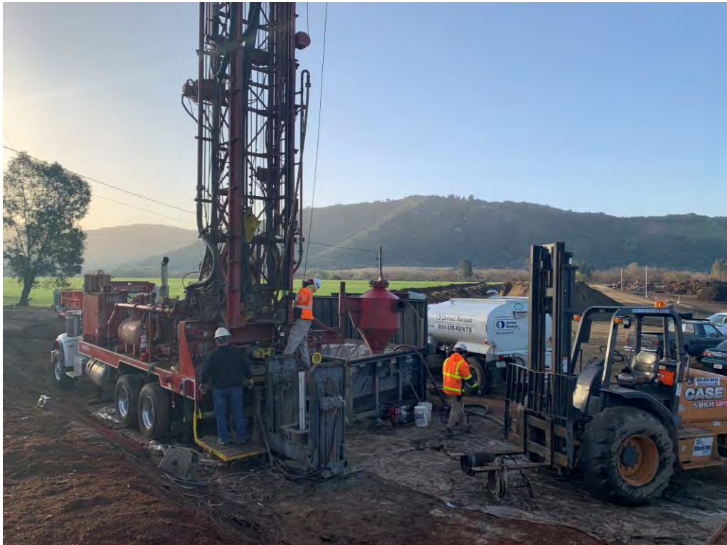
Photograph 6 - ARCH drill rig set up at SP129, during well installation.
