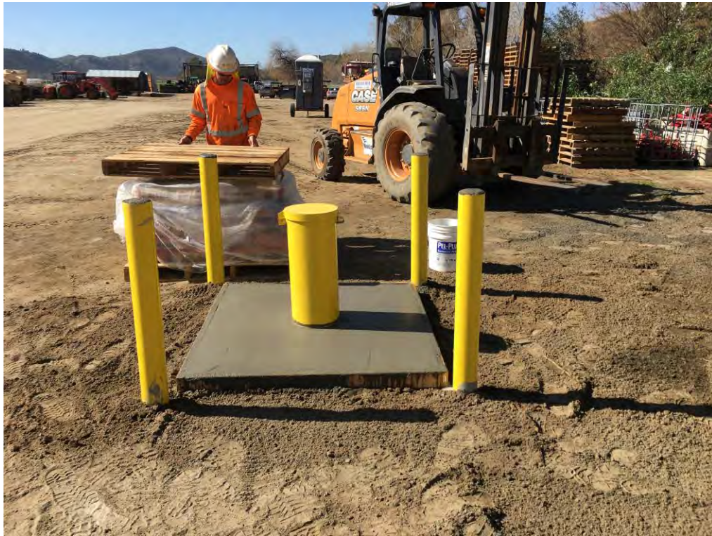
Photograph 5 - SP128 surface completion.
