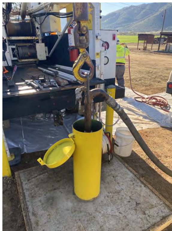
Photograph 8 - Air lift piping during well development.
