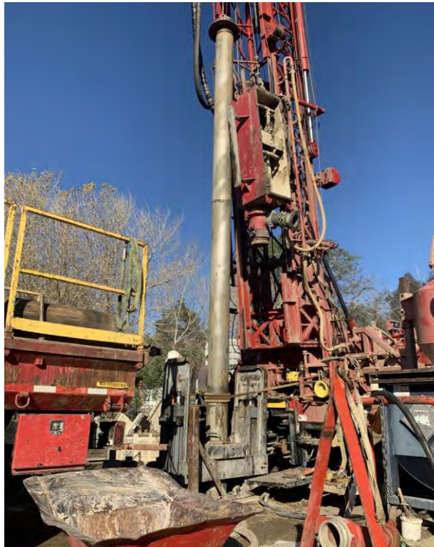
Photograph 4 - Removing conductor casing at SP128 during well installation.
