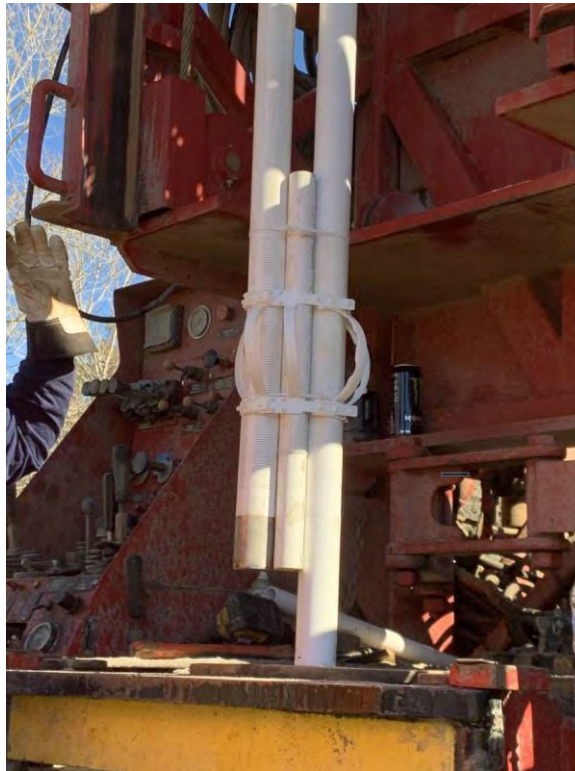
Photograph 3 - Well installation at SP128.
