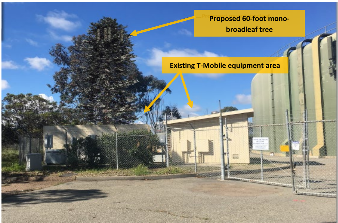
Figure 2: Photo-simulation of proposed Verizon mono-broadleaf and existing equipment shelter.
