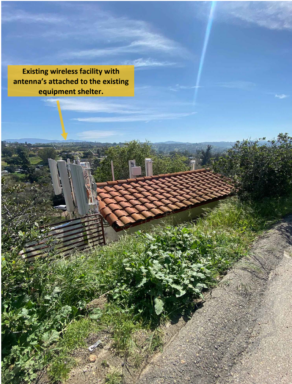
Figure 1: Existing Southeast view of 15.6-foot-tall wireless facility with equipment located on and within a 180 square feet equipment shelter.
