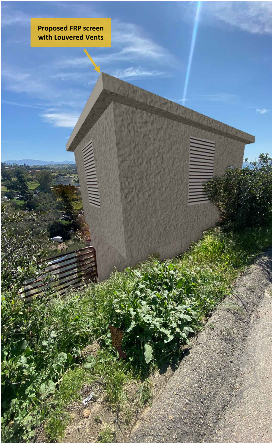
Figure 2: Proposed Southeast view of 18-foot-tall wireless facility with equipment located within a 180 square foot FRP screened equipment shelter.
