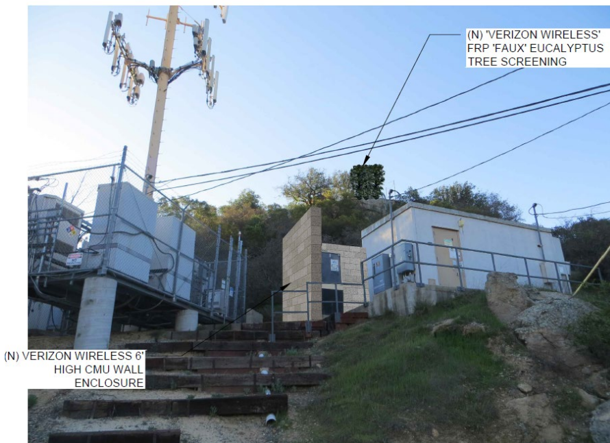
Figure 2: A 6-foot-tall CMU wall is proposed to enclose the facility's backup generator and the northern portion of the equipment shelter within the 360-square-foot leased area.
