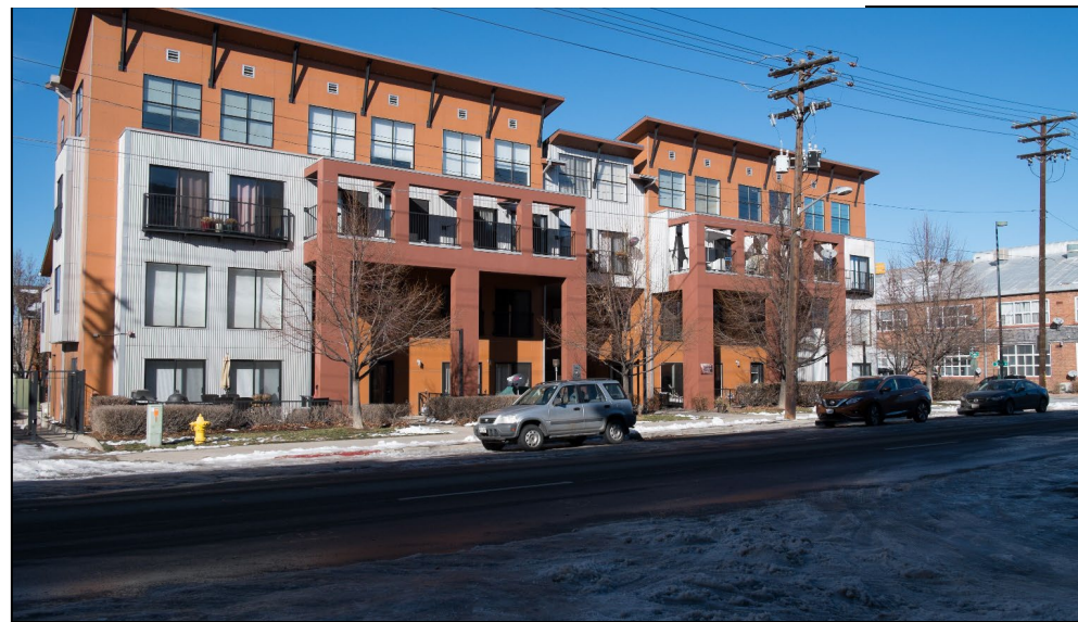
Figure 2-14: Infill Development - Denver, Colorado
