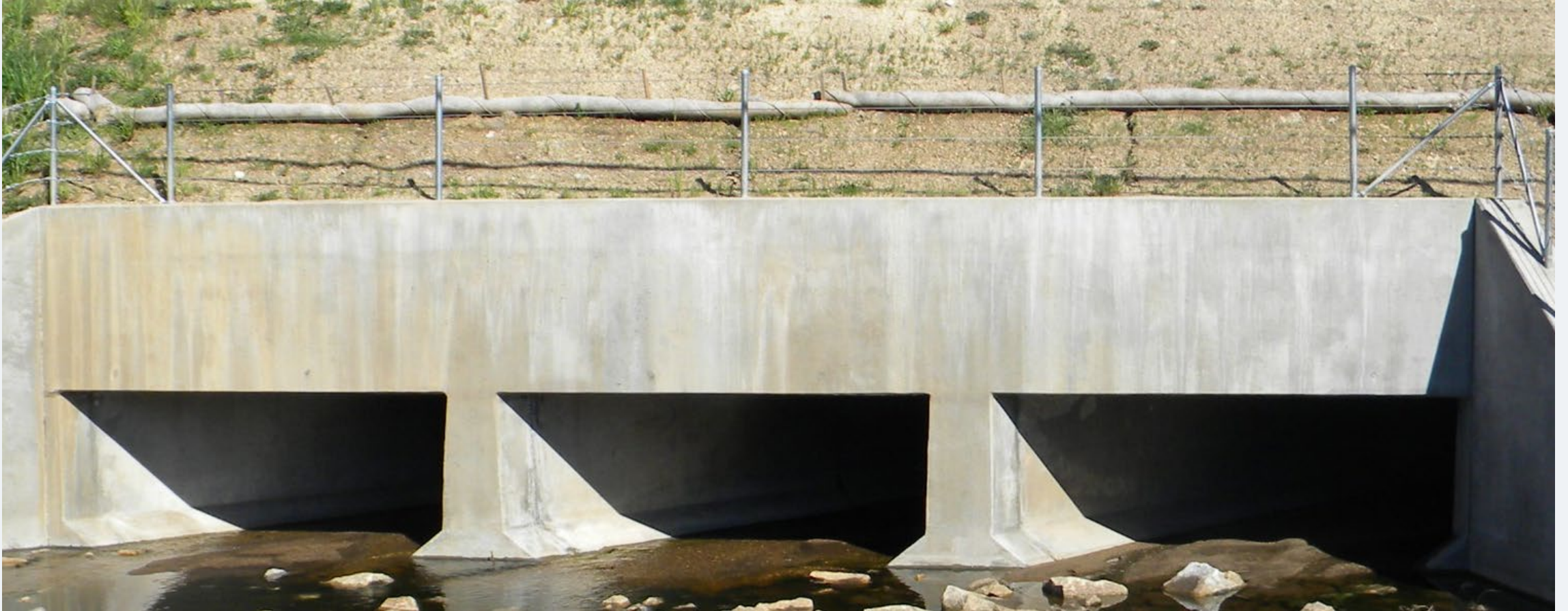
Picture: Example of drainage culverts
