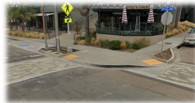
Figure 12: Curb extensions at Camino Del Mar & 12 th Street in Del Mar
