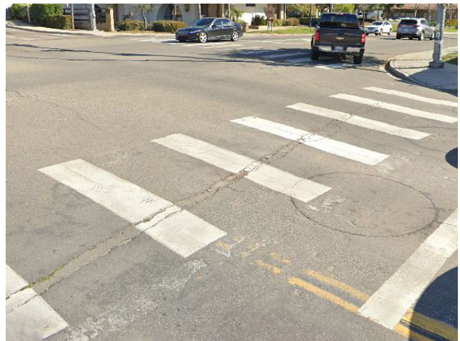
Example of a continental crosswalk in Fallbrook at Fallbrook Street and Main Avenue
