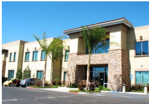
Office complex in Rancho San Diego
