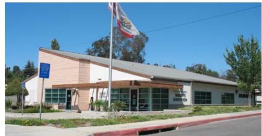
Fallbrook Sheriff substation
