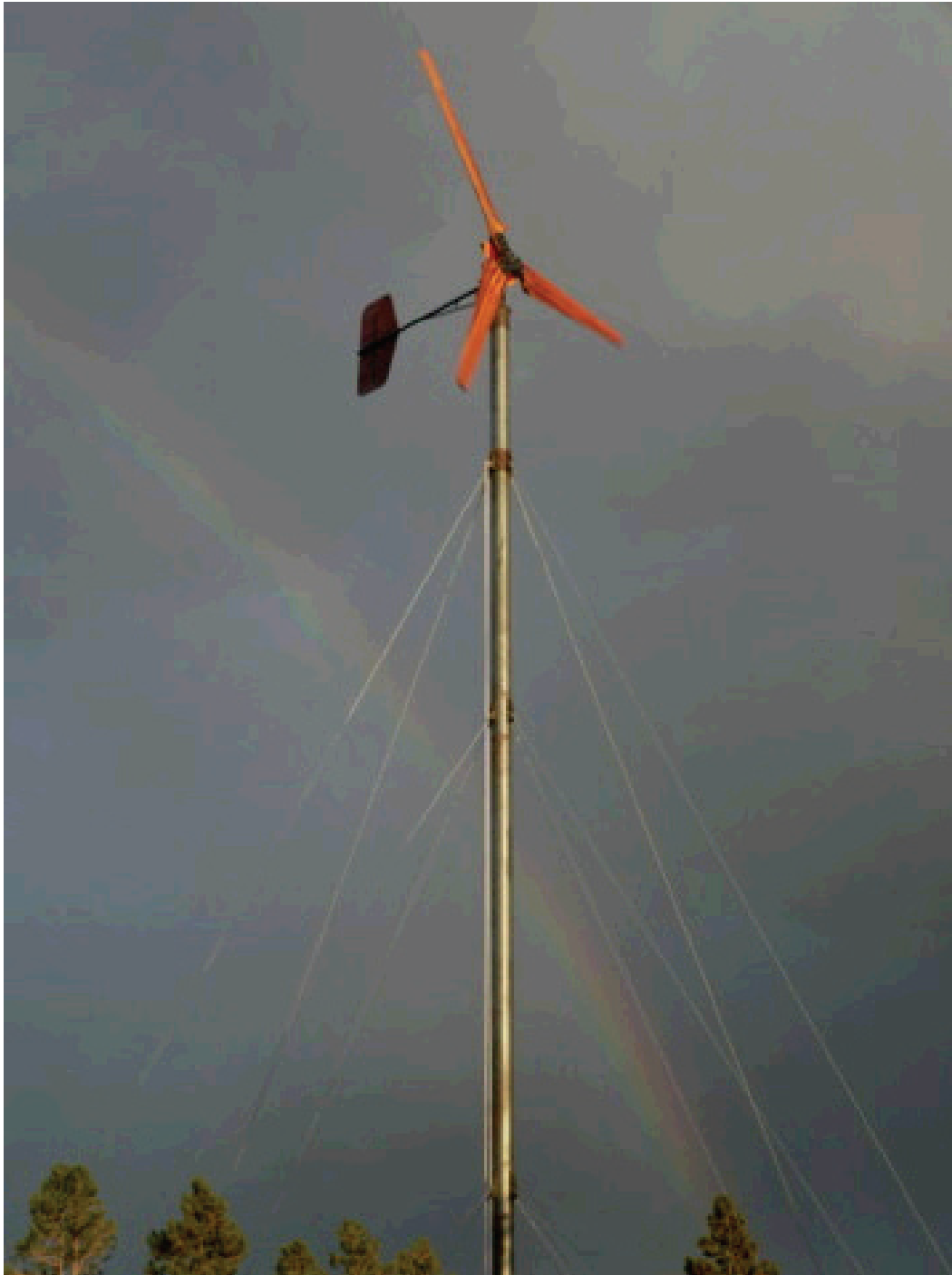
Guywire Monopole Structure
