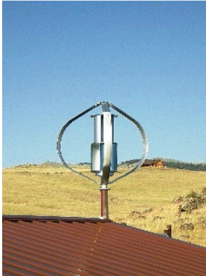
Roof Mounted Vertical Axis Turbine
