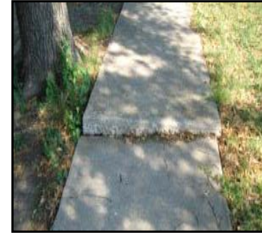
Surface roots have raised the sidewalk.
