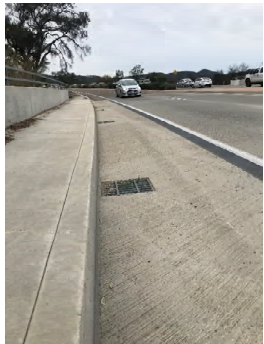
Figure 20: Class II bike lane with drainage inlet.
