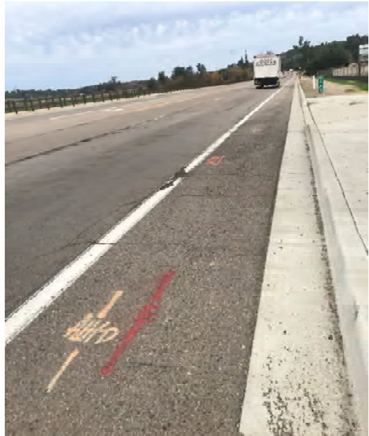
Figure 19: Class II bike lane with degraded surface.
