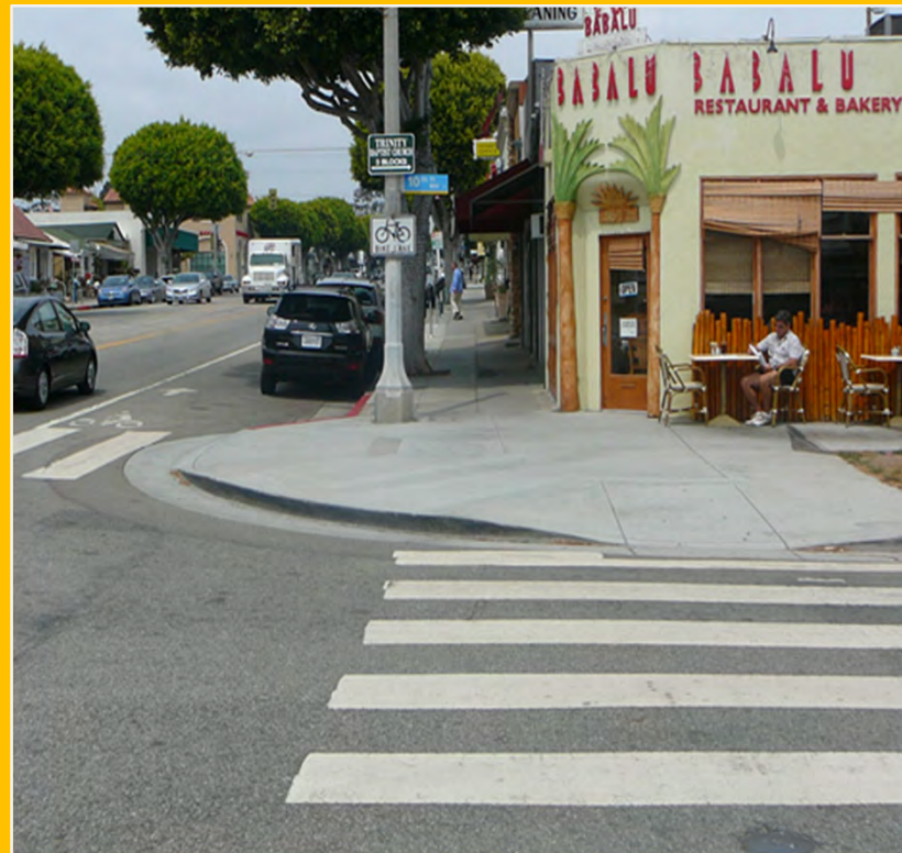
Curb-Extensions at Intersection
