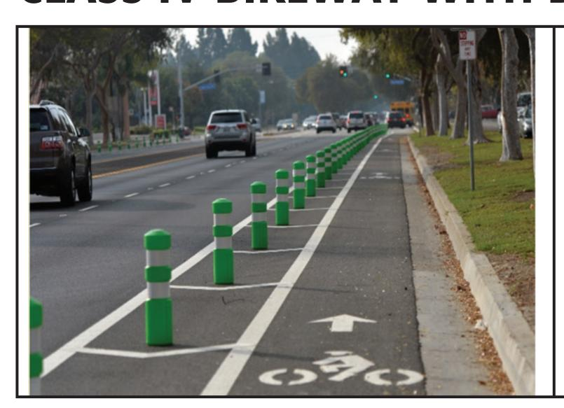
Provides a physical separation between bicycles and moving traffic
