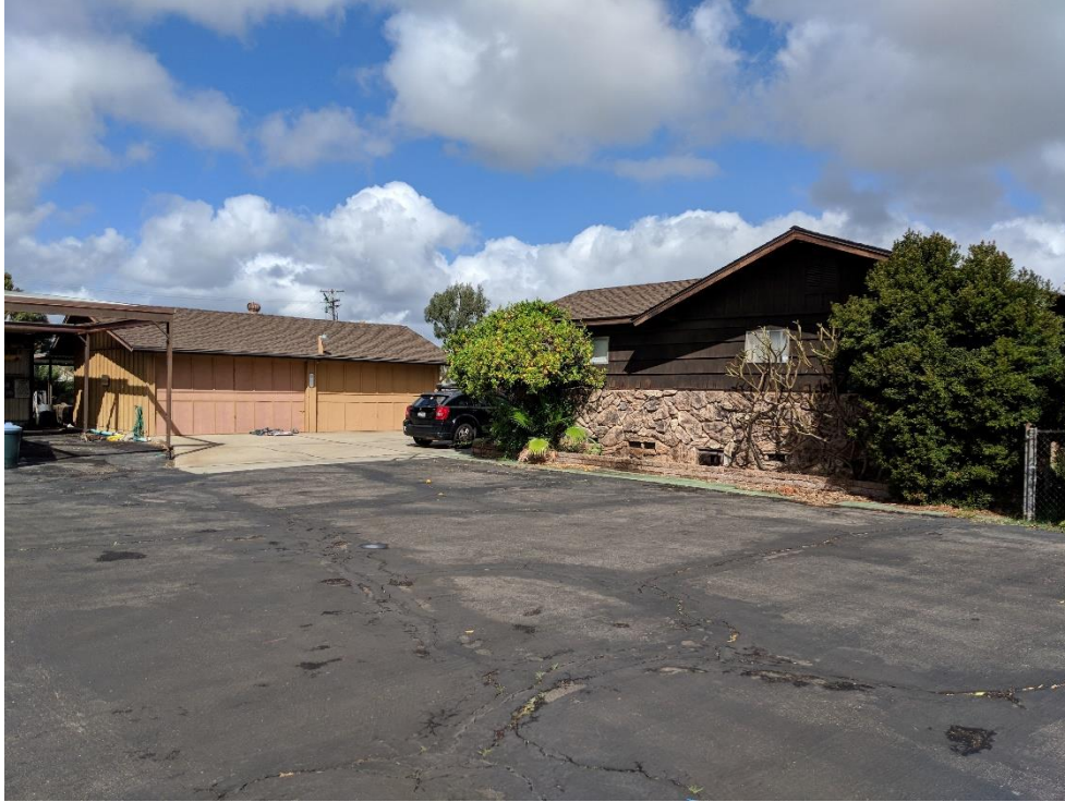
Figure 1. 1118 N Anza St - RV port, garage, and S side, facing NW; 3/15/2018
