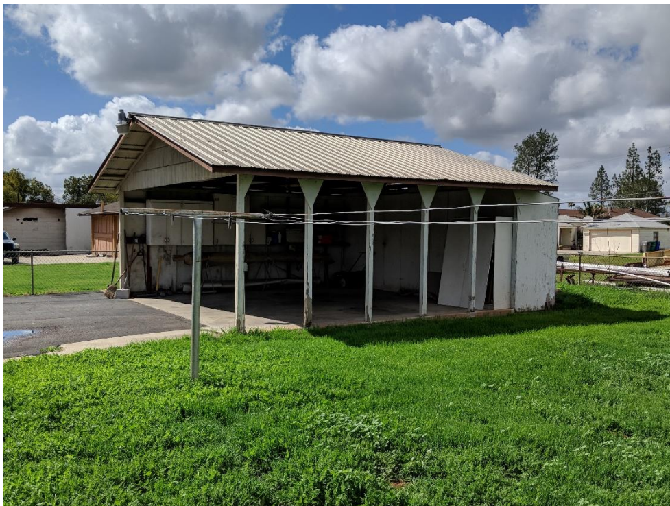
Figure 2. 1132 N Anza St - garage, facing SW; 3/15/2018
