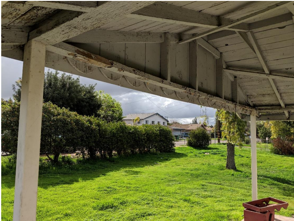
Figure 2. 1112 N Anza Street interior front porch, facing SE; 3/15/2018
