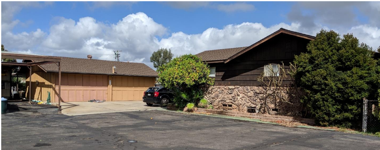
Figure 6. 1118 N Anza Street house and garage, facing northwest; 3/15/2018
