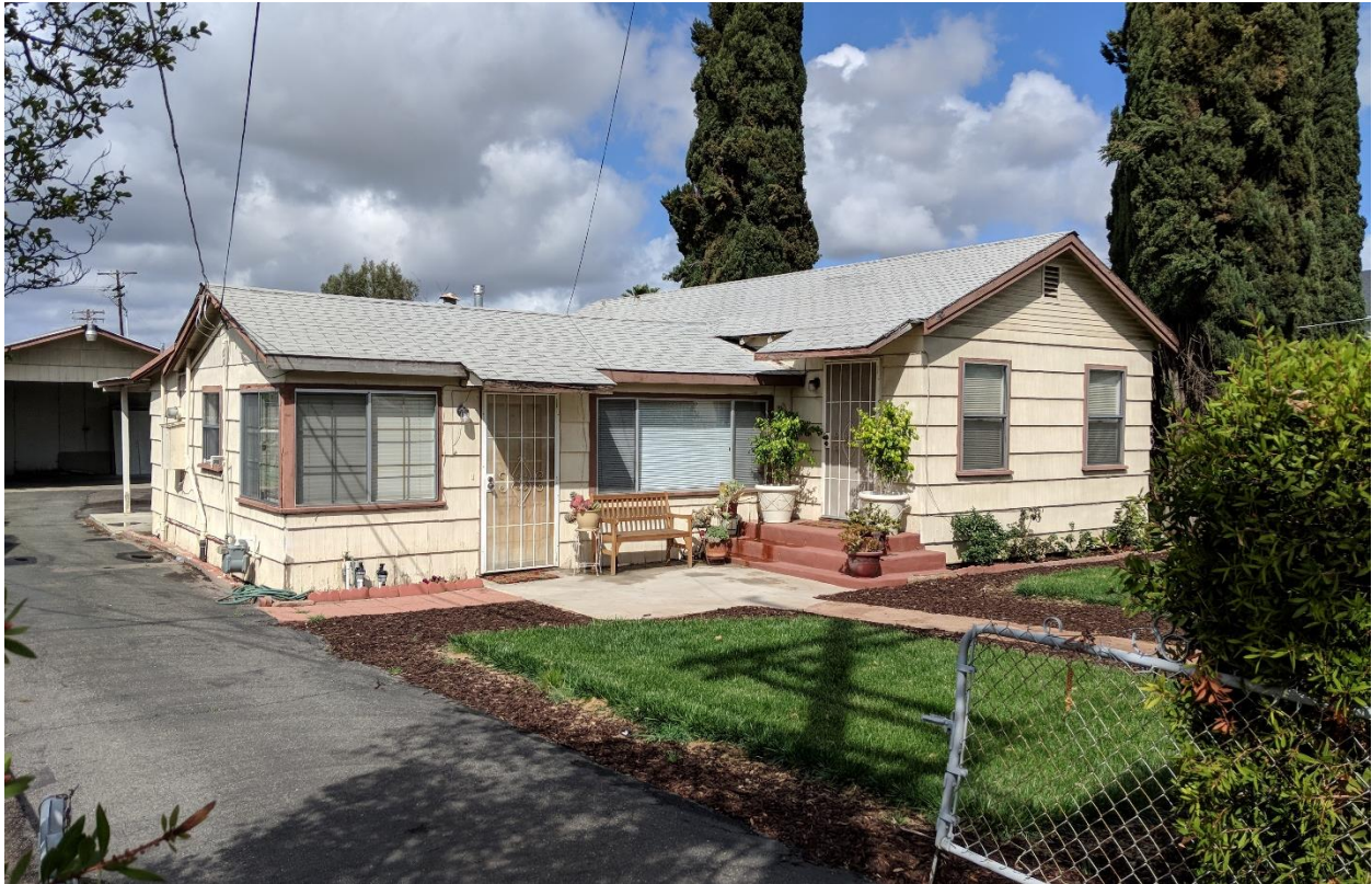
Figure 7. 1132 N Anza Street house and garage, facing northwest; 3/15/2018
