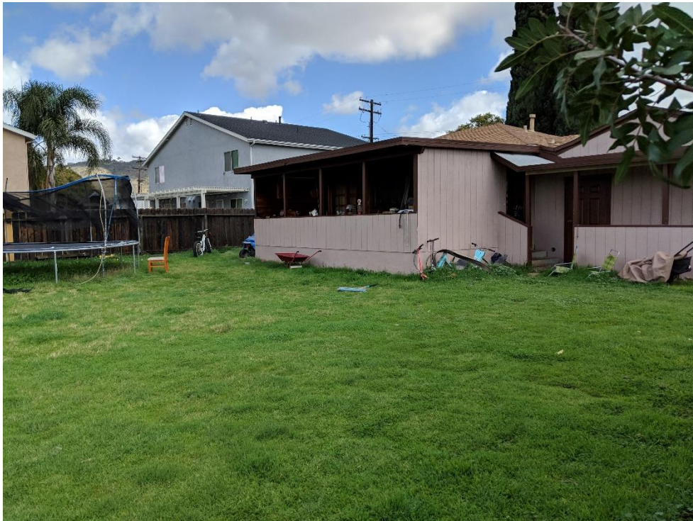
Figure 2. 1136 N Anza St - back extension, facing NE; 3/15/2018
