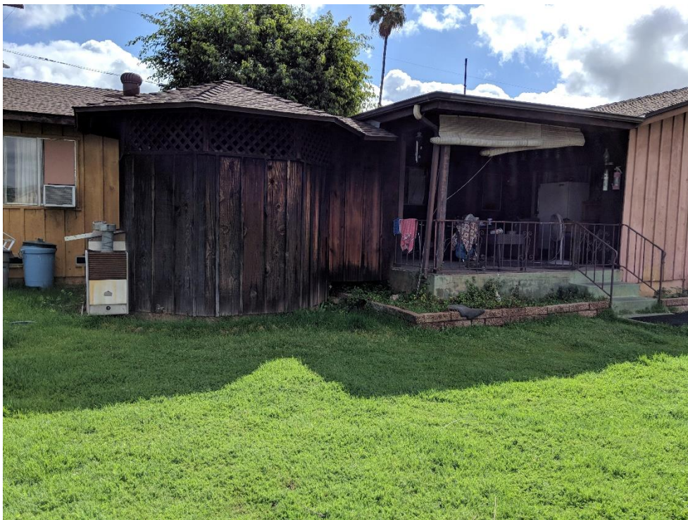
Figure 2. 1118 N Anza St - rear view, facing east; 3/15/2018
