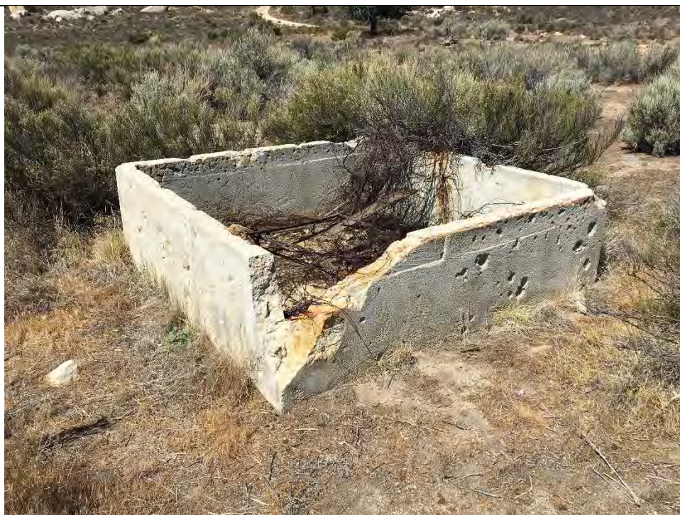
Photo 31. Possible cistern 5' x 5' and about 2' tall. Broken glass, wood planks and metal wiring inside.
