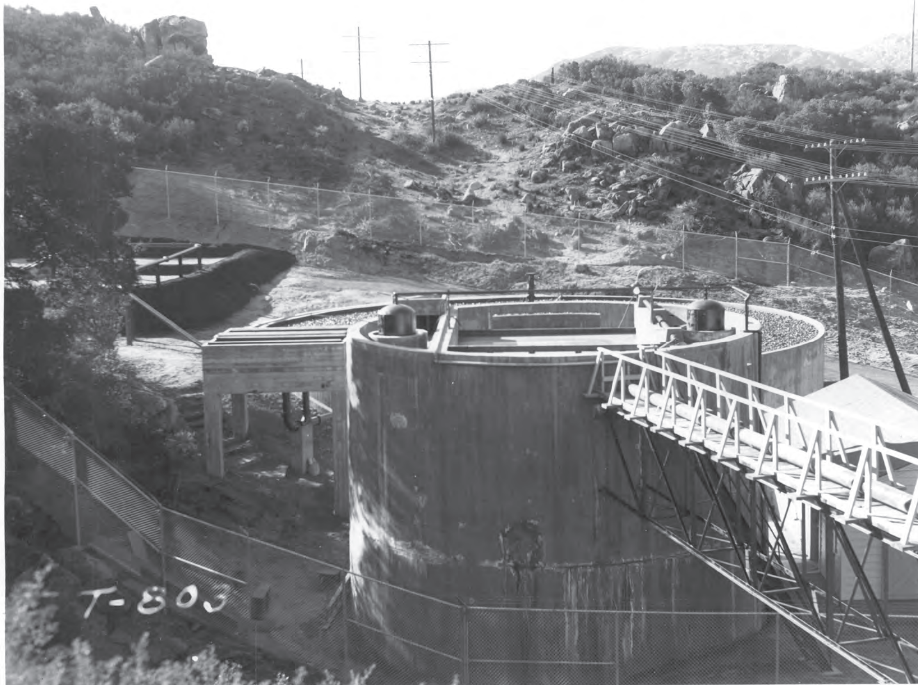
Imhoff Tank; Sewage Disposal Plant
