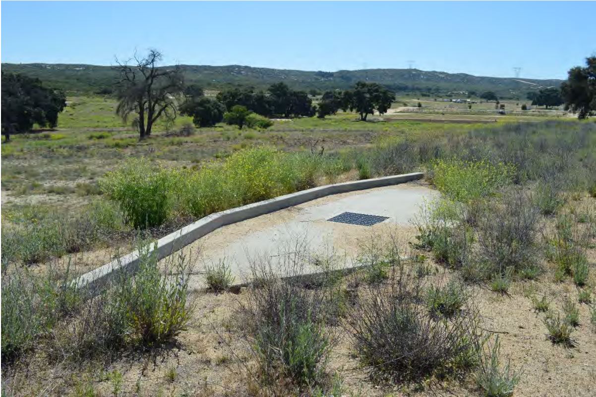
Figure 40. Concrete Drainage Structure, Center of Running Track
