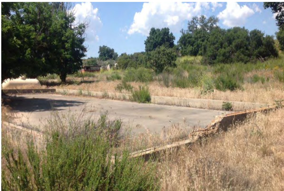
Figure 77. Historic Foundation Slab with New Poured Concrete
