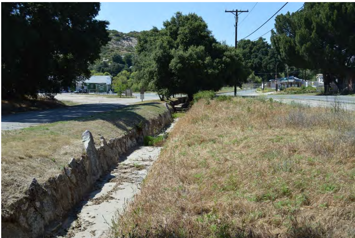
Figure 35. Stone-Lined Portion of Main Ditch near Entrance Area
