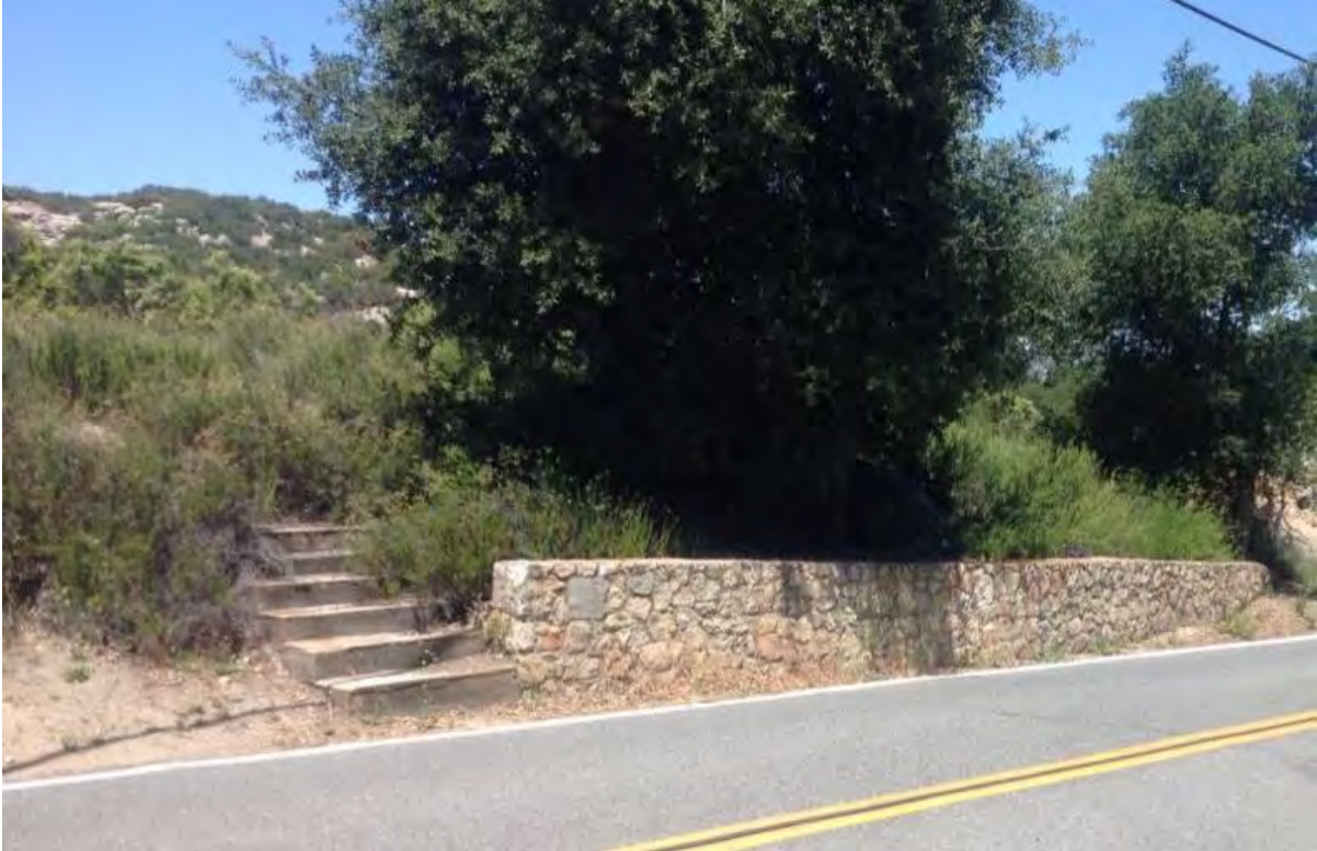
Figure 71. Mortared Granite Wall
