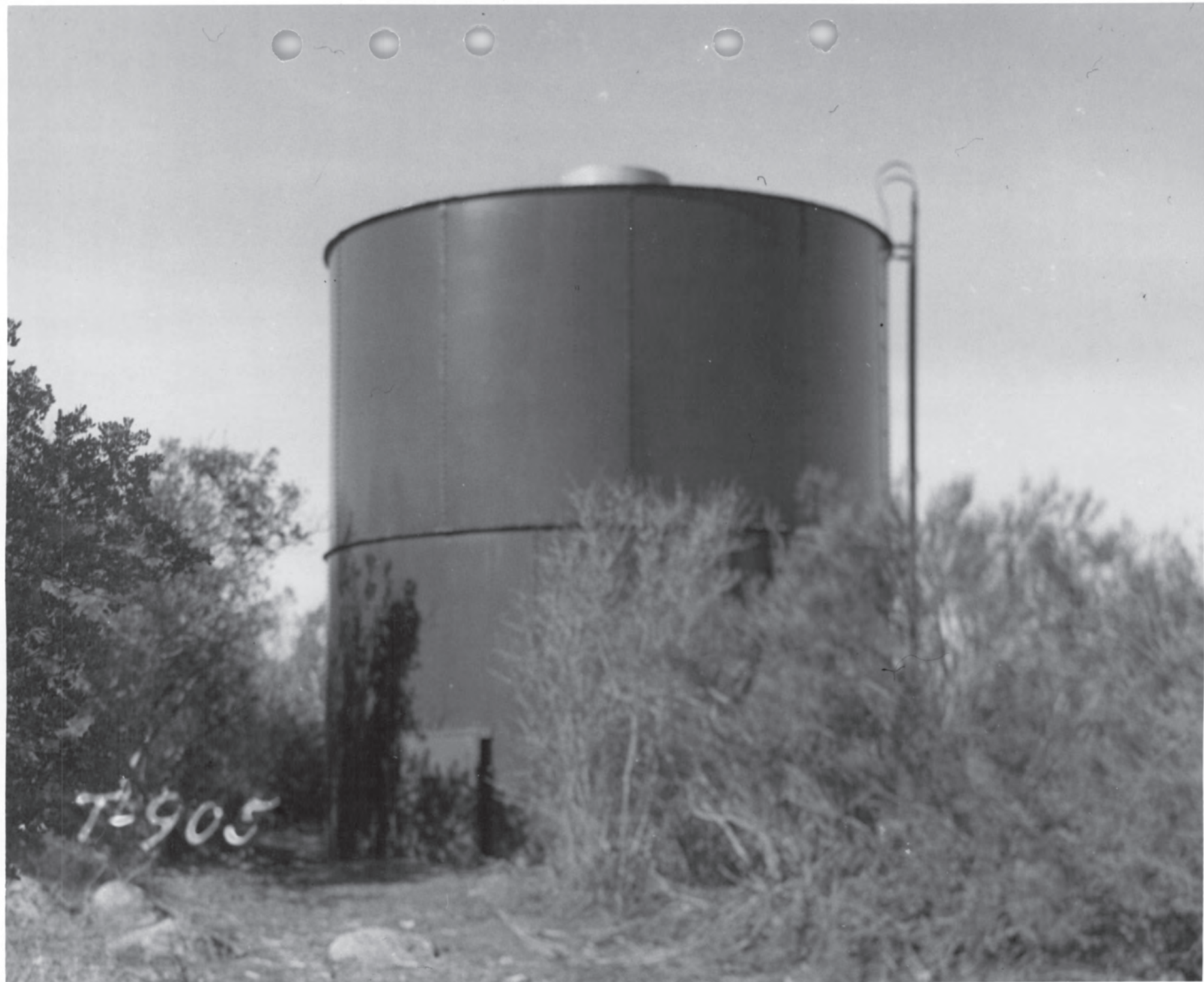
Backwash tank; Morena Water Supply System
