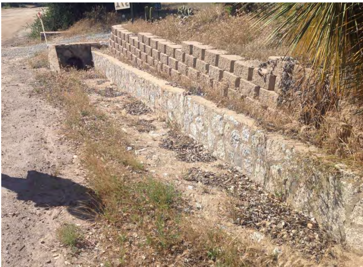
Figure 37. Mortared Rock Walls and Ditches, North Side of Moore Road
