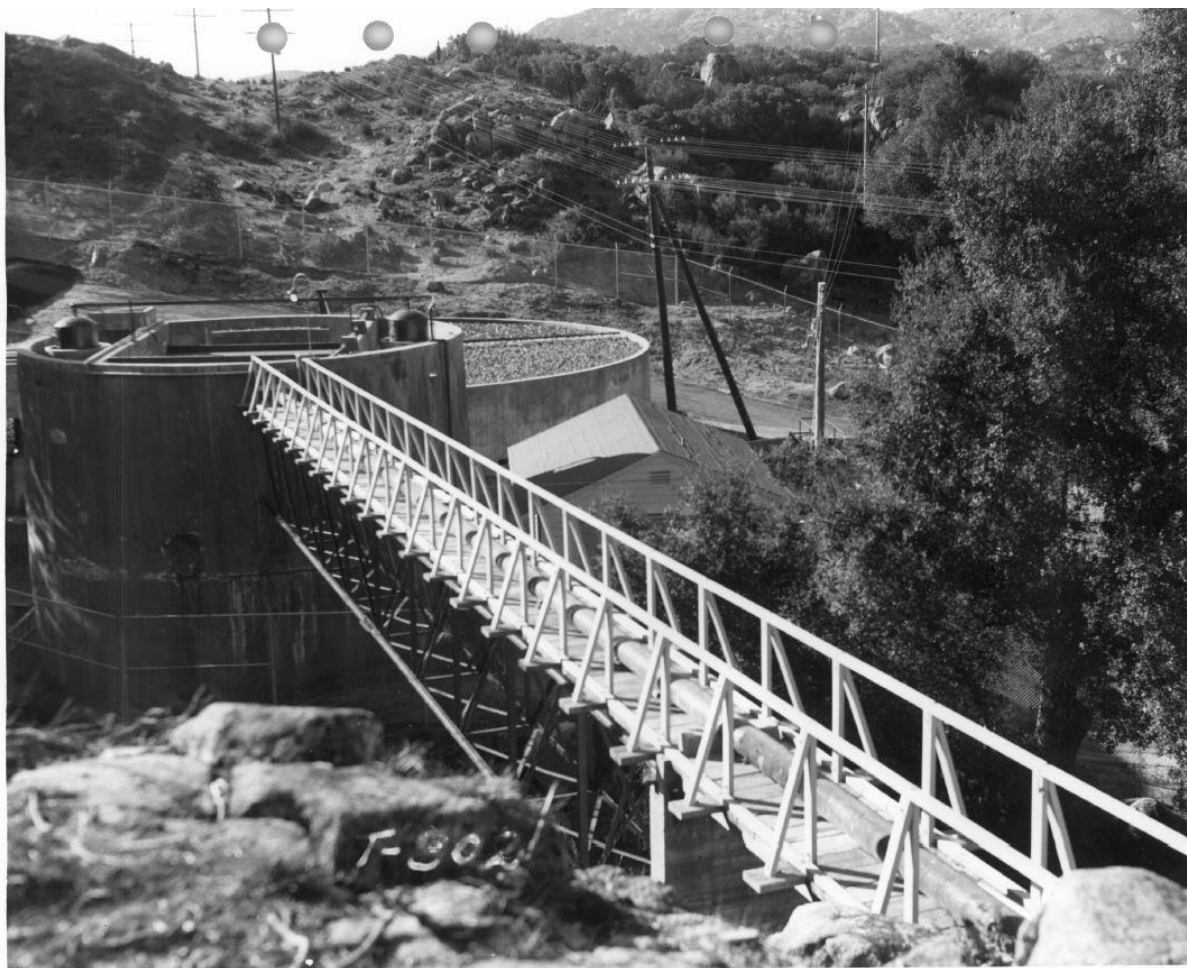
Figure 36. Trestle and Flume Connecting Sewage Treatment Plant and Camp
