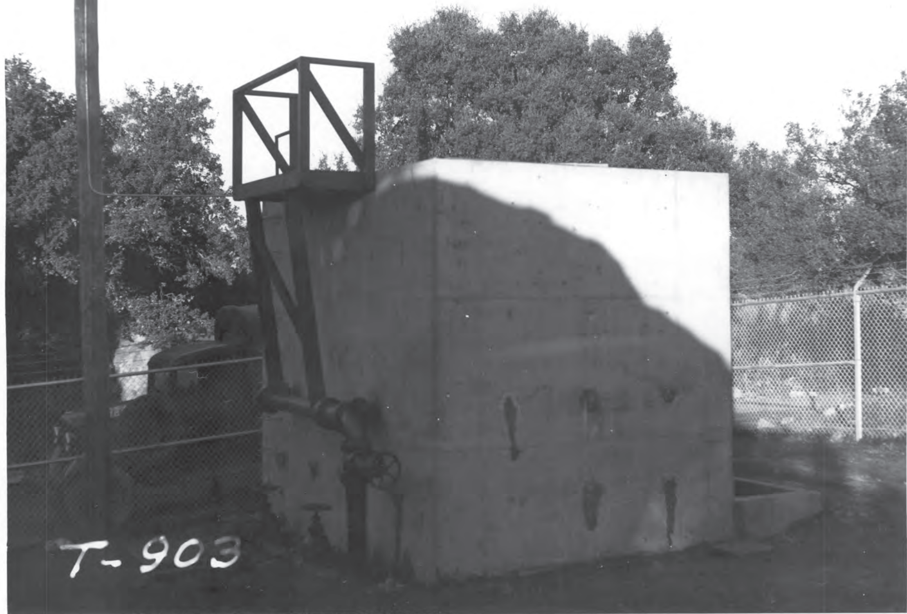
Sand Filter, Korena Water Supply System
