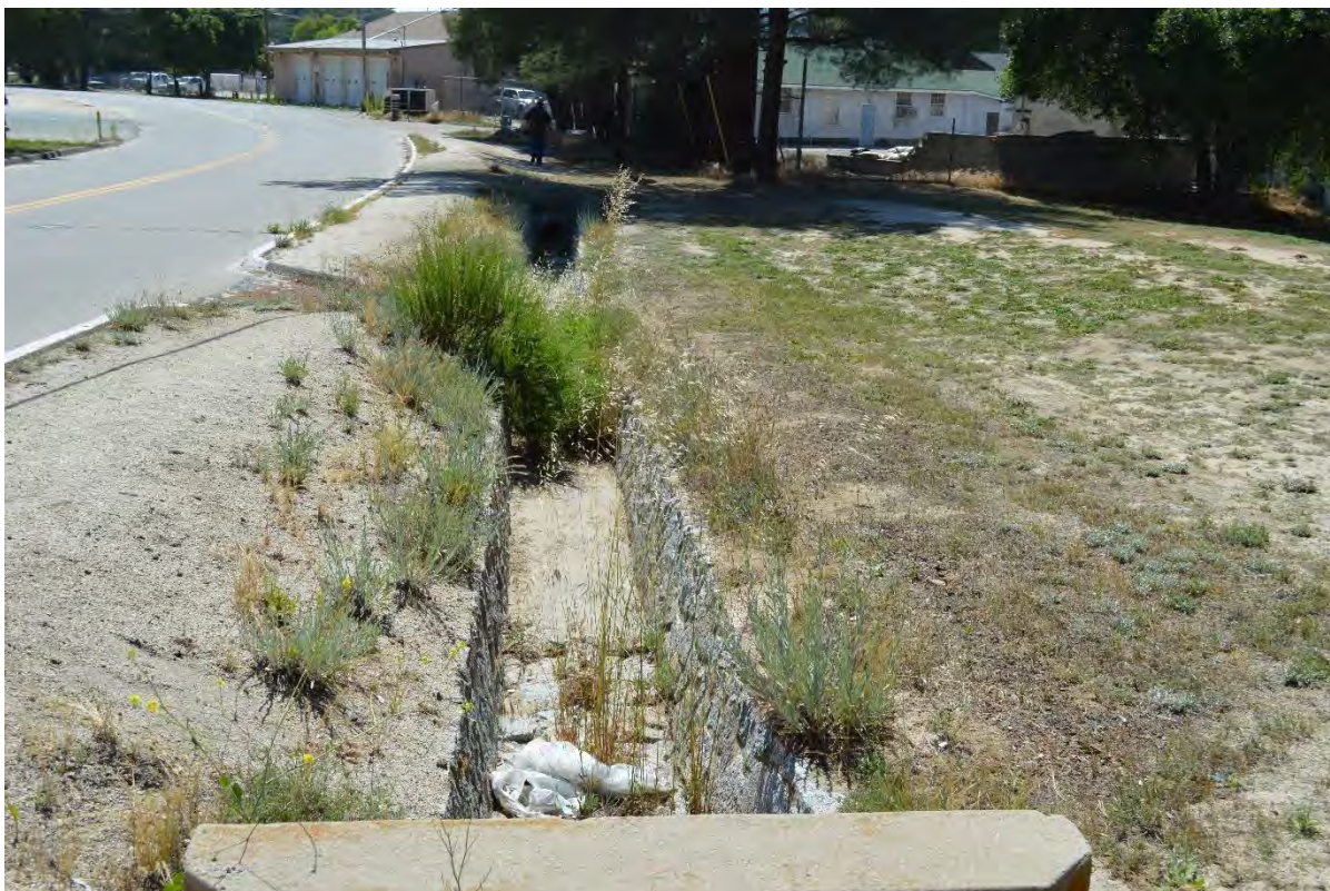
Figure 34. Stone-Lined Drainage Ditch along Jeb Stuart Road
