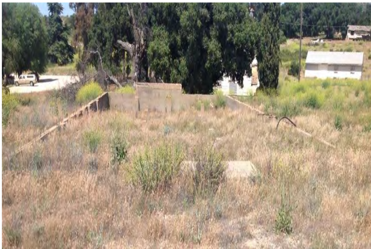
Figure 75. Chapel Foundation West of Theater with Concrete Piers Chapel foundation west of theater with concrete piers in the center. Source: ICF June 2019.
