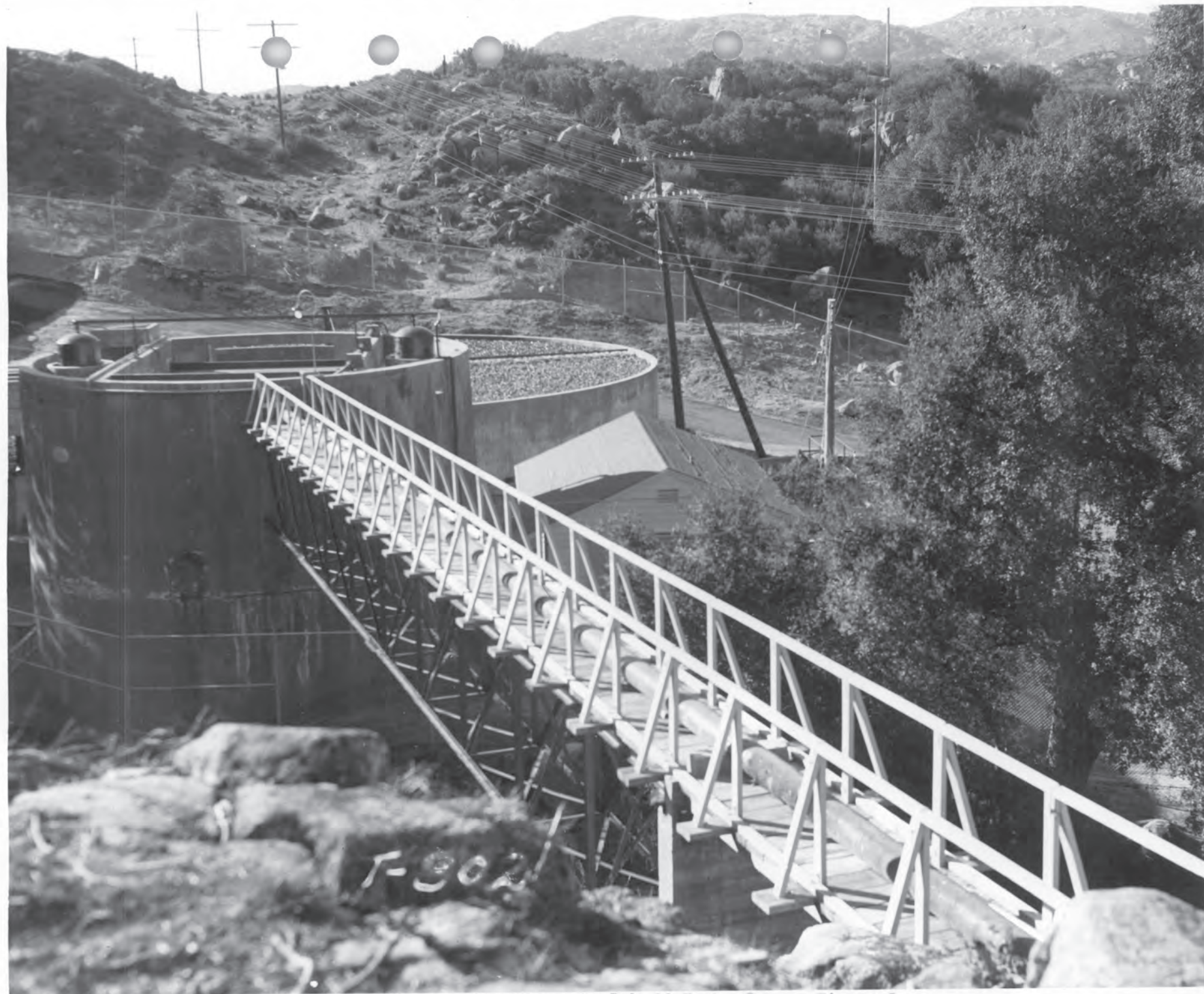
Trestle, Palmer-Bowlus Flume to Imhoff Tank, Sewage Disposal
