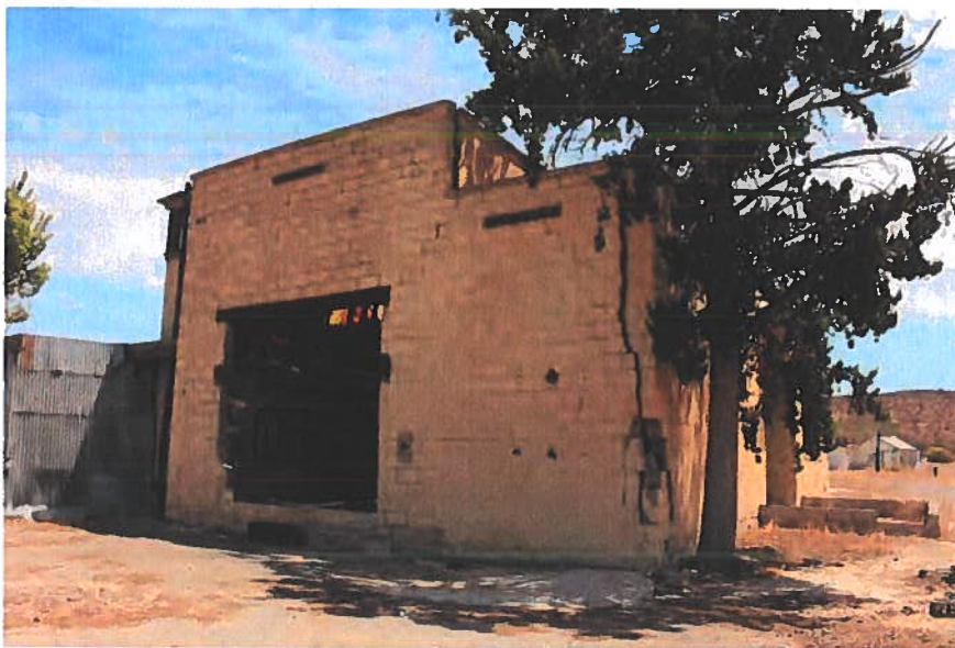
Figure 2. Detail of Structural Failure Tank House West Elevation, 2018.
