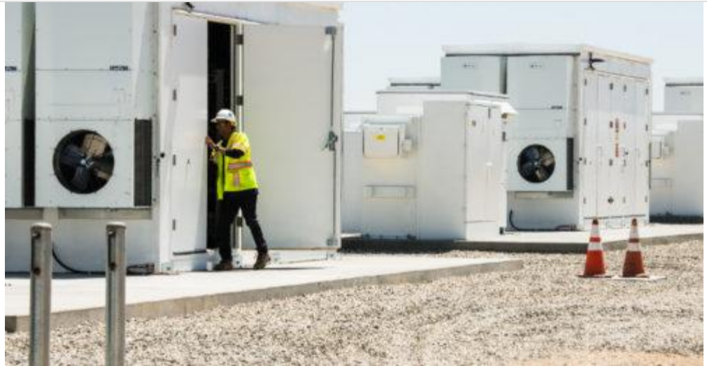
This large-scale lithium battery installation in California shows the ventilation systems used to keep batteries at a consistent temperature to prevent thermal runaway. (Photo by Dennis Schroeder / NREL)
