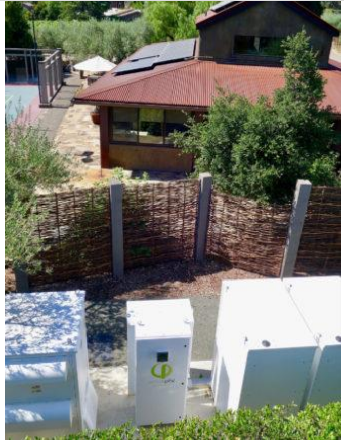
This LFP battery with inverter charge controllers, power electronics and system management was installed in a NEMA 3R outdoor-rated box, away from livable spaces, just in the off-chance of an accident.
