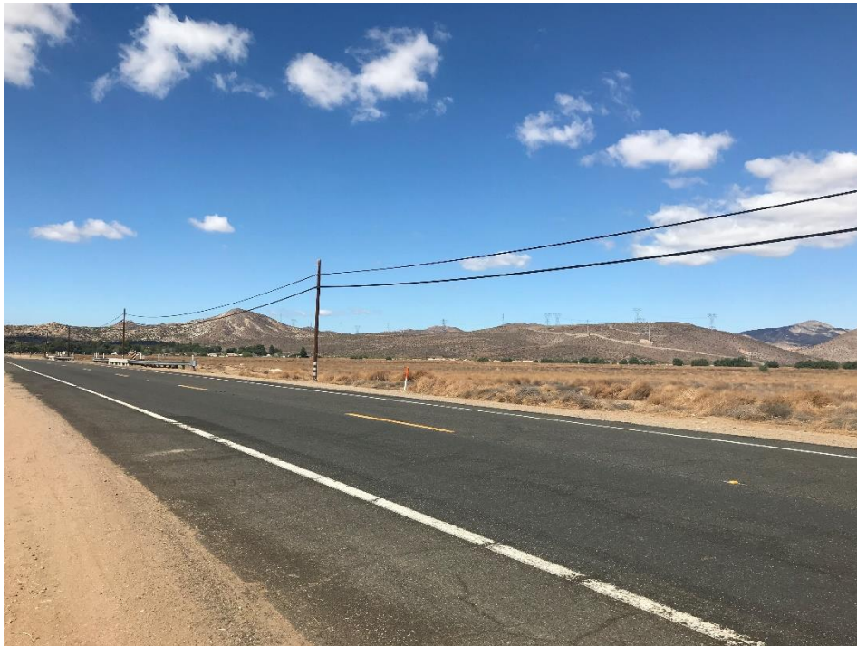
Key View 2: View northwest from westbound Old Highway 80
