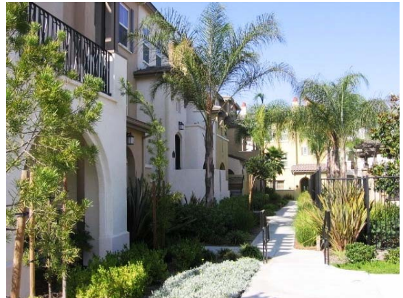
Multi-family housing units in 4S Ranch
