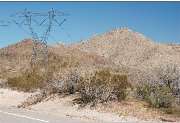
Photo 2 - Southwest Power Link (SWPL) Poles 210-213. Demonstrating that under certain lighting conditions the open lattice nature allows the structures to be less visually prominent when they are not skylined
