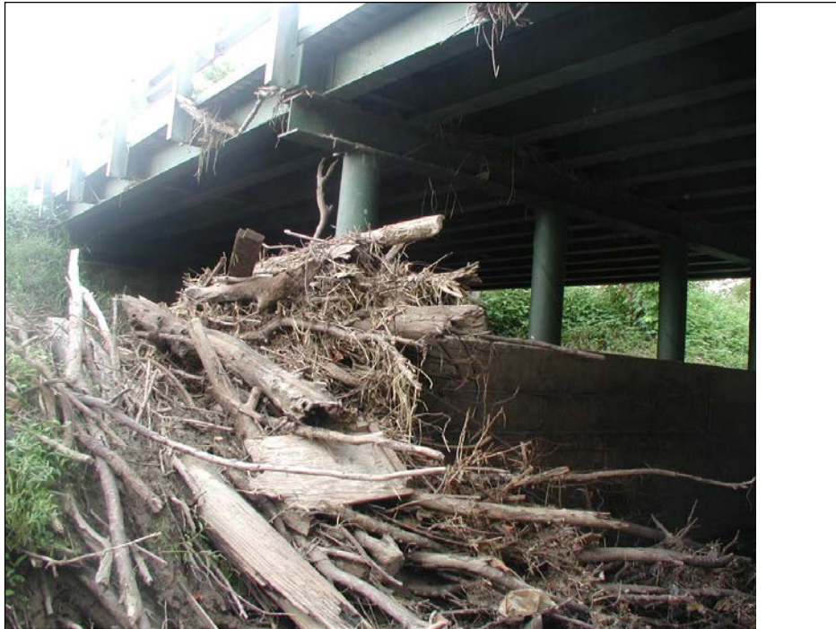
Figure 7.15. Woody debris at a bridge pier. Note how debris can be much wider than the pier itself (also note debris on lower chord of bridge deck). Source: NCHRP Web-Only Document 48 (see NCHRP 2010a).
