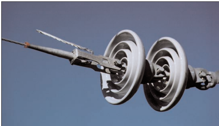
Figure 3-68 Automatic Deadends with Suspension Insulators
