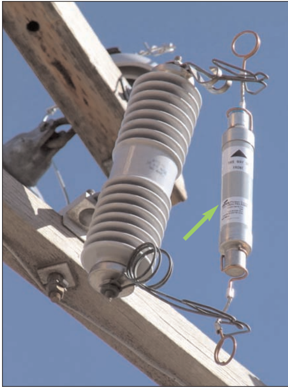
Figure 3-6 Also Fits "Open Link" Cutouts
