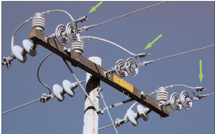
Figure3-48 Parallel Groove Connectors on Jumpers
