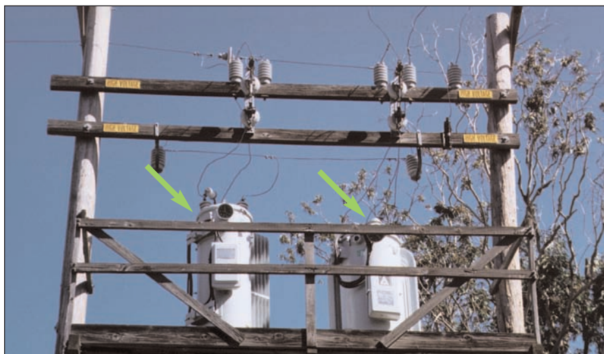
Figure 3-41 Voltage Regulator
