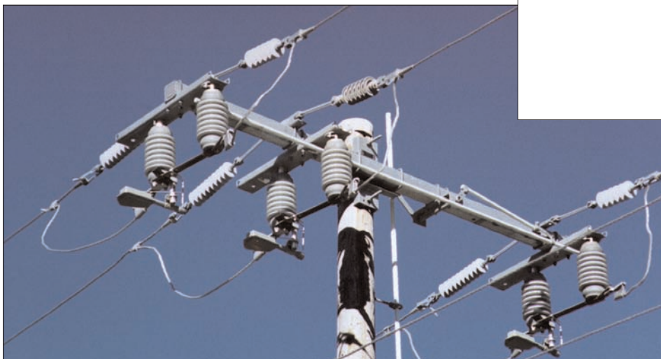
Figure 3-27 600 Amp Underarm Sidebreak Switch (closed position))
