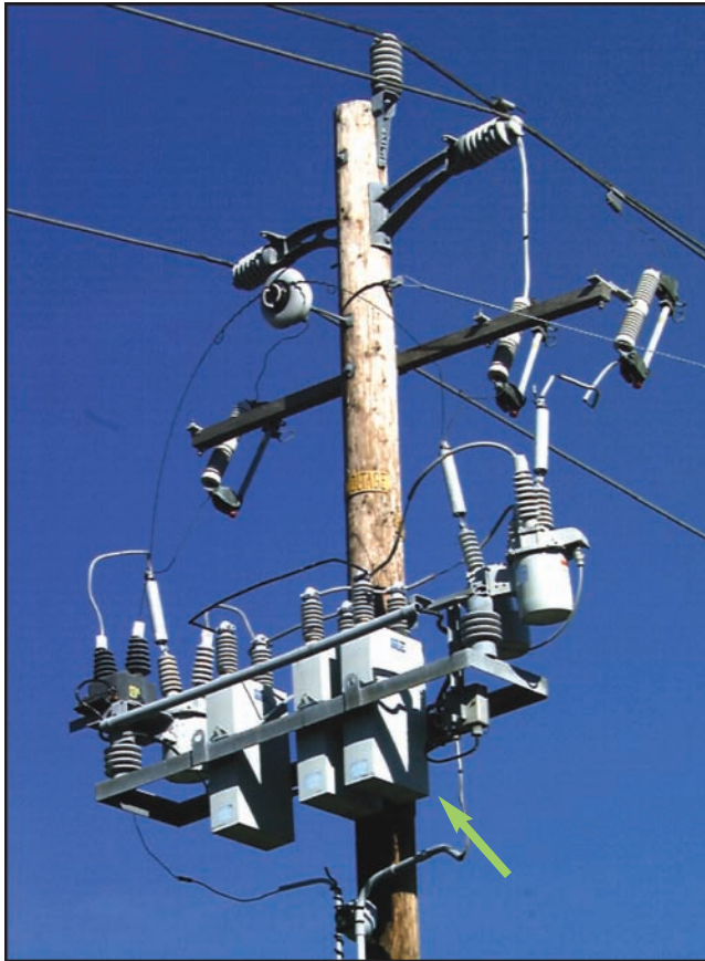
Figure 3-42 Capacitor Bank
