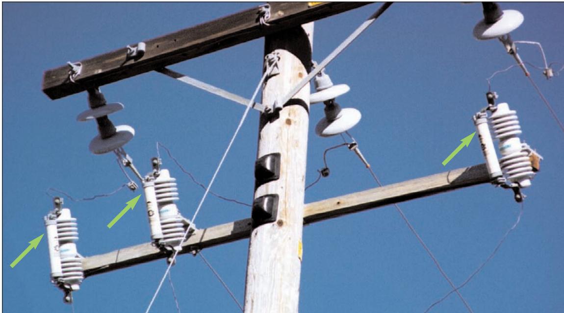
Figure 3-3 Arm Mounted Cutout with Non-Expulsion Fuses
