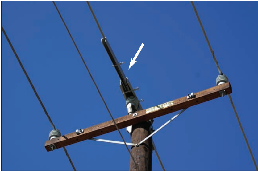
Figure 4-22 Raptor Protector Insulator and Wire Cover
