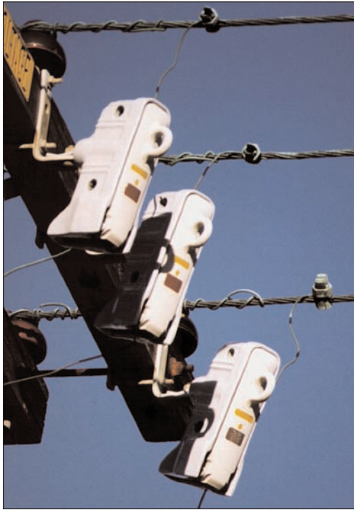
Figure 2-8 Enclosed Cutouts
