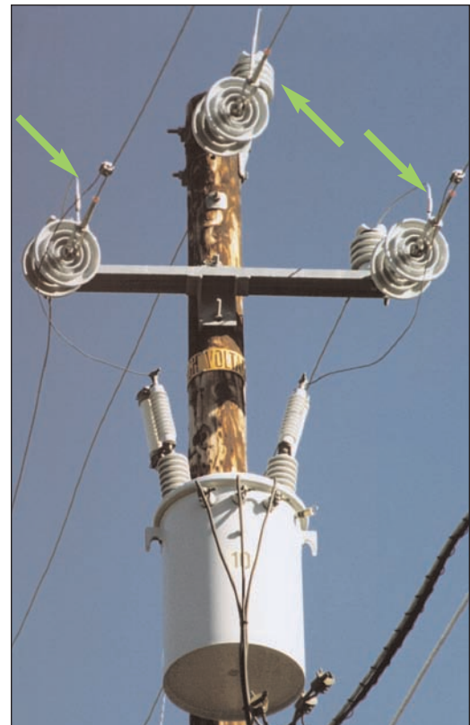
Figure 3-69 Automatic Deadends Attached to Pole and Crossarm
