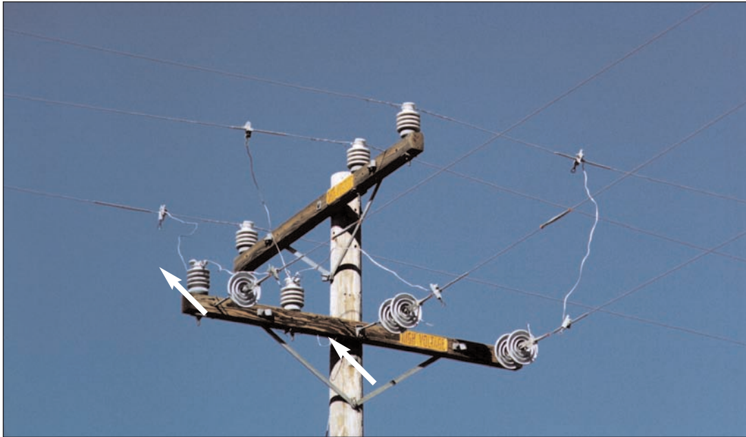
Figure 4-5 Tangent Crossarm with Deadend Tap (T-Tap)
