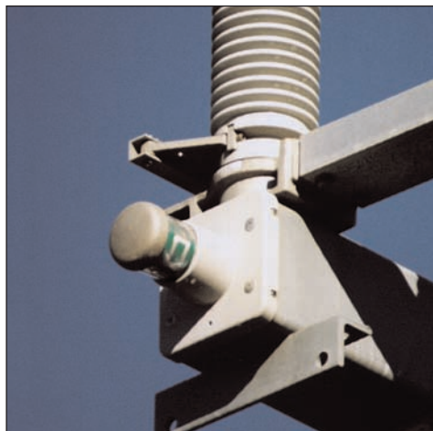
Figure 3-34 Open Position Indicator Green Letter "O" visible
