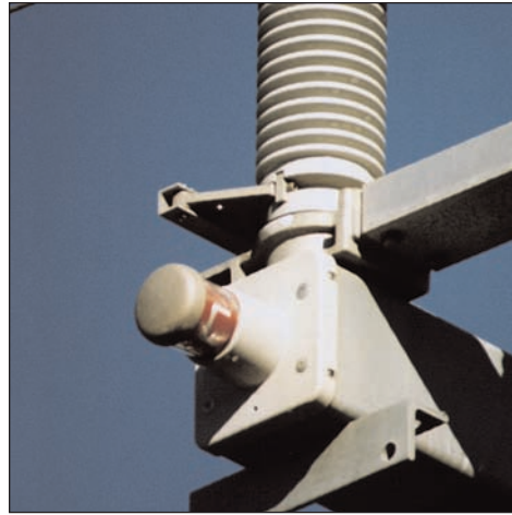
Figure 3-35 Closed Position Indicator Red
