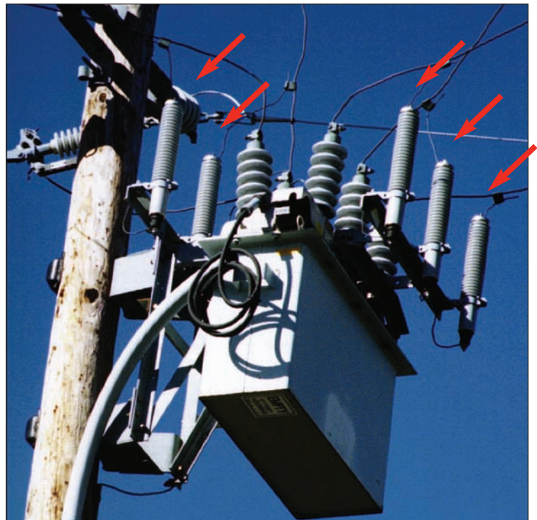
Figure 2-20 Lightning Arrester (with Recloser)
