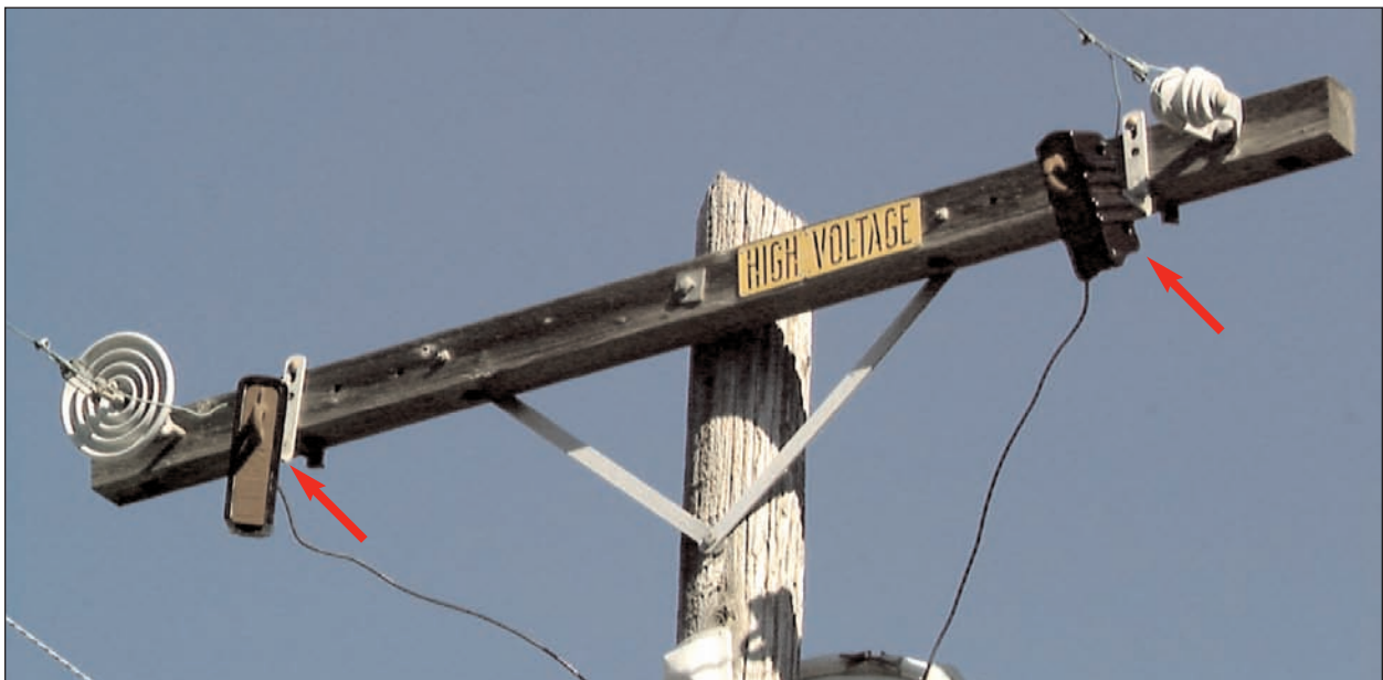
Figure 2-10 Arm Mounted Enclosed Cutout with Universal Fuses
