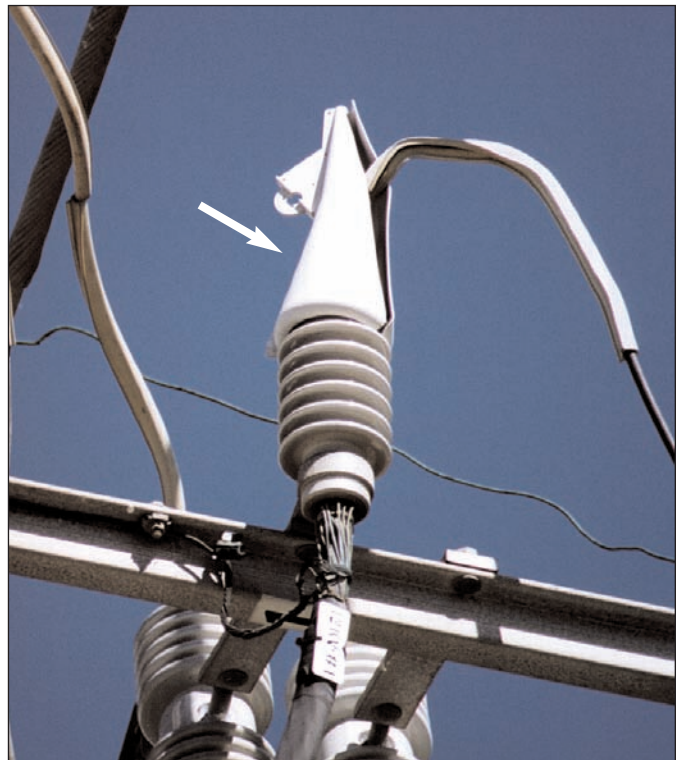
Figure 4-21 Close up of Squirrel Guard
