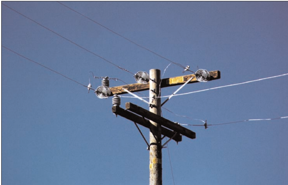
Figure 4-6 Crossarm Deadend Corner (Line and Buck)
