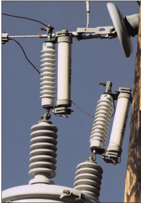
Figure 3-4 Bushing Mounted Cutout with Non-Expulsion Fuse
