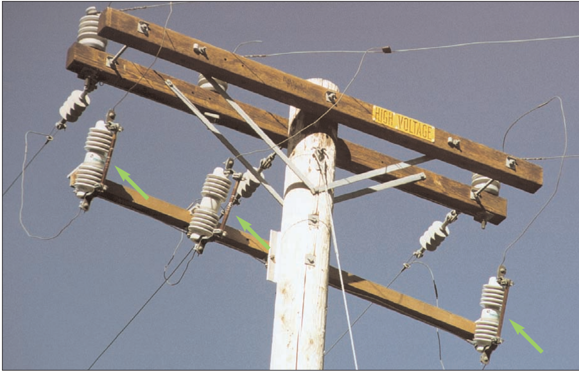
Figure 3-10 Arm Mounted Cutout with Liquid Filled Fuse
