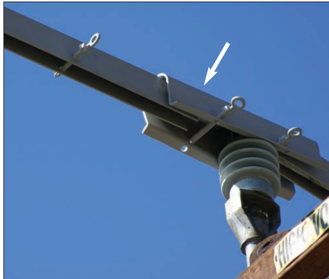
Figure 4-23 Close up of Insulator and Wire Cover
