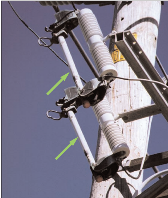
Figure 3-14 Arm Mounted Cutout with SMU-20 Fuses
