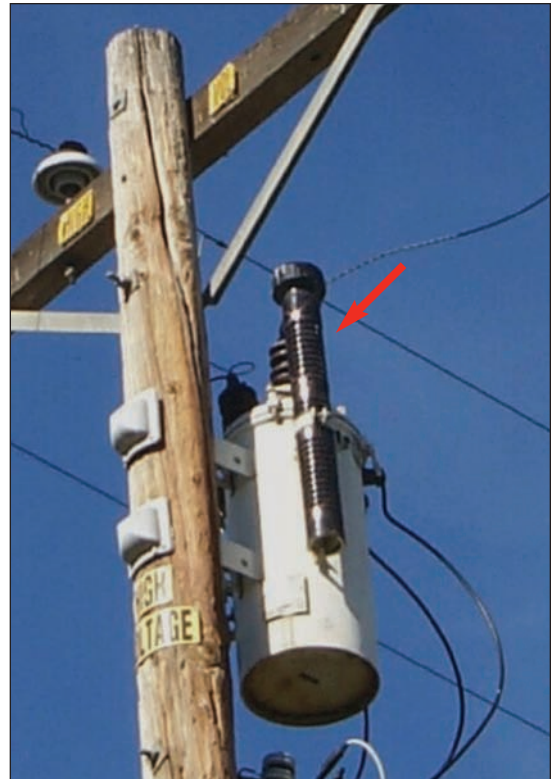
Figure 2-28 Lightning Arrester
