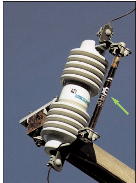
Figure 3-11 Liquid Filled Fuse
