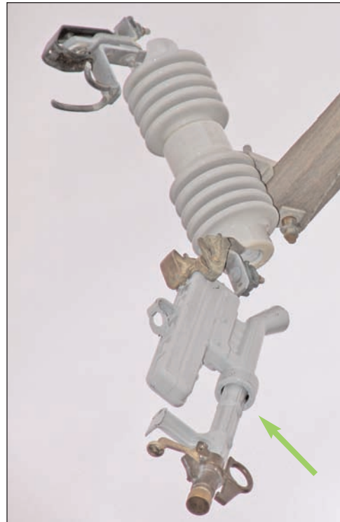
Figure 3-19 S&C Fault Tamer Fuse (Open)
