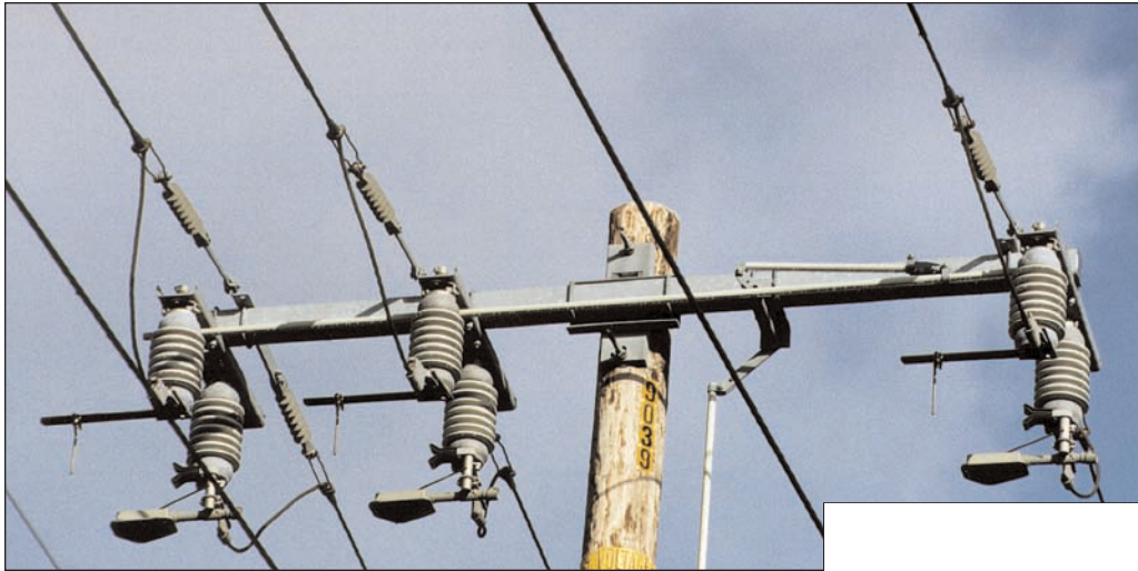
Figure 3-24 600 Amp Underarm Sidebreak Switch (open position)
