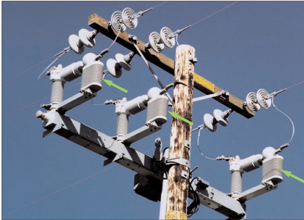
Figure 3-33 S&C Scada-Mate Switch
