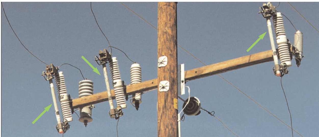
Figure 3-16 Arm Mounted Cutout with SMU-20 Fuses
