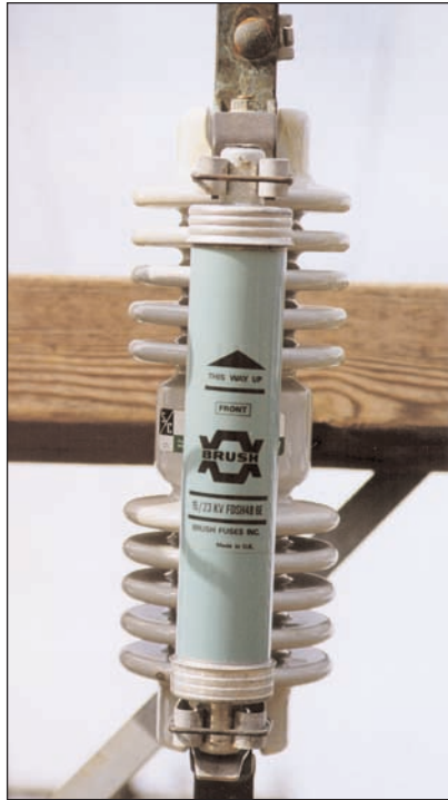
Figure 3-2 Arm Mounted Cutout with Non-Expulsion Fuse
