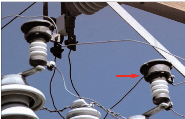
Figure 2-22 Lightning Arrester
