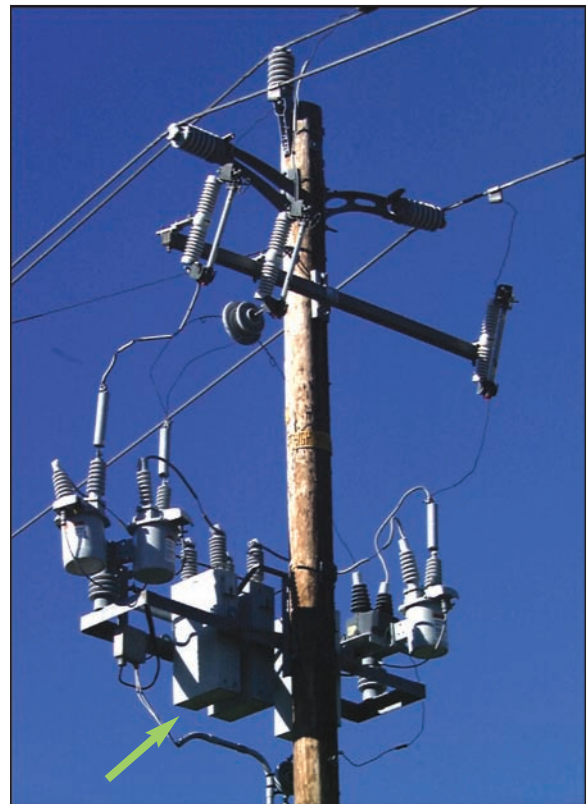
Figure 3-43 Capacitor Unit
