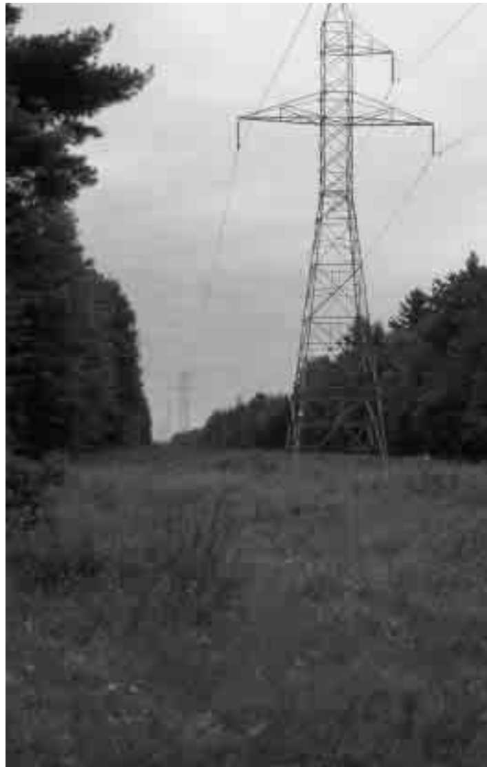
Fig. 4–3 Transmission line clearings are examples of disturbance corridors that are maintained by continued human intervention. Near Ottawa, southern Ontario, Canada. (Photo: A. Bennett).
