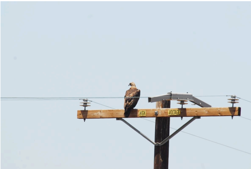
A male Golden Eagle from the Bandy Canyon territory hunting from telephone poles north of the Ramona Airport; 2009. Note the raptor guard placed by SDG & E over the center conductor.
