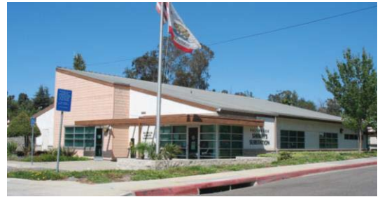
Fallbrook Sheriff substation
