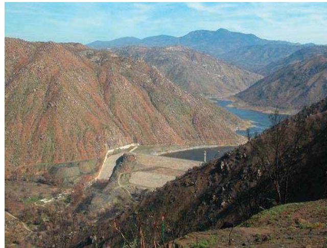
Dam in unincorporated County
