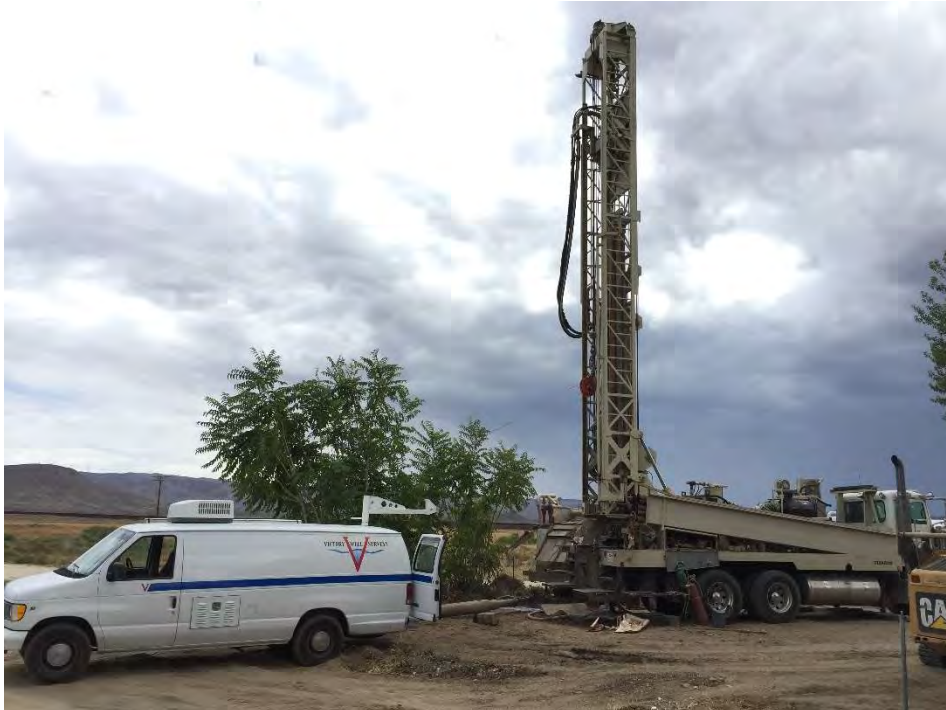
Photograph 2. Victory Survey geophysical logging pilot borehole.
