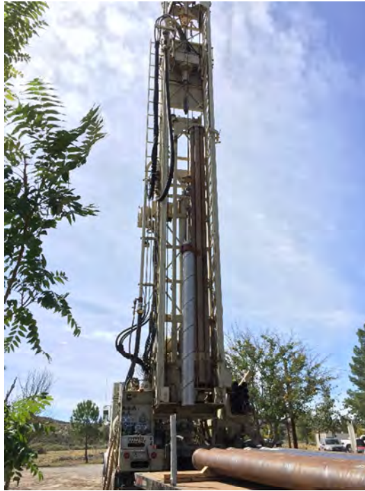
Photograph 13. Installation of 10 foot stainless steel sump.
