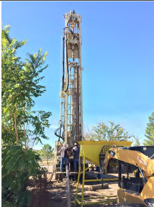
Photograph 10. Installing 2-inch diameter tremie pipe.
