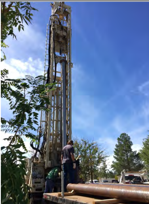
Photograph 14. Installation of stainless steel well screen.
