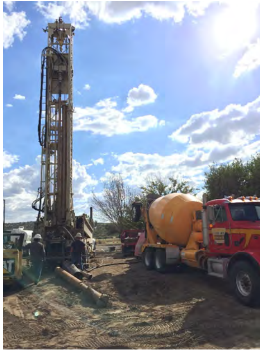
Photograph 5. Setting 50 foot sanitary cement seal, 10.3-sack cement slurry.
