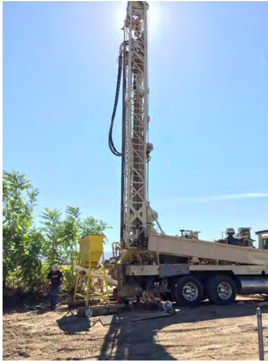
Photograph 11. Tremie silica sand into borehole.
