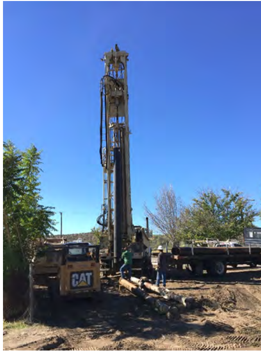
Photograph 3. 16-inch diameter steel conductor casing installation.
