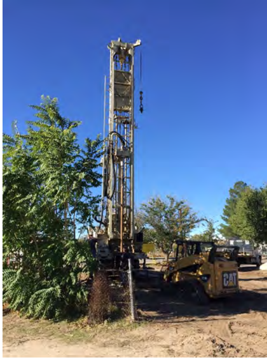
Photograph 9. Fain performing a cleaning pass before casing installation.
