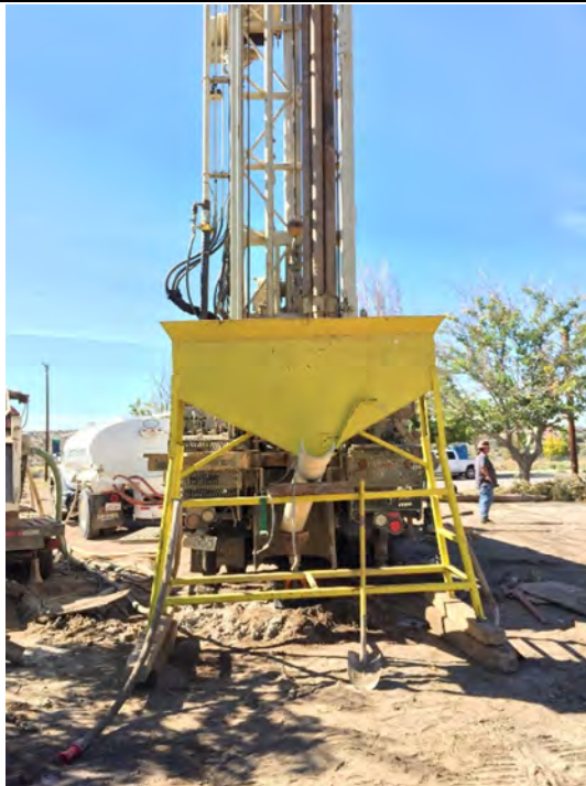
Photograph 12. Hopper feeding silica sand into tremie pipe.
