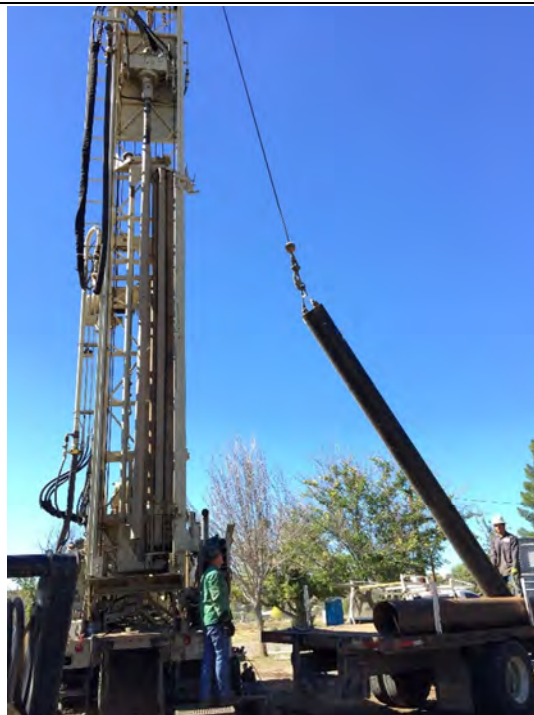
Photograph 4. 16-inch diameter steel conductor casing installation.
