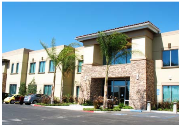
Office complex in Rancho San Diego
