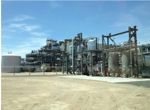
Figure 4. Power generation building.
