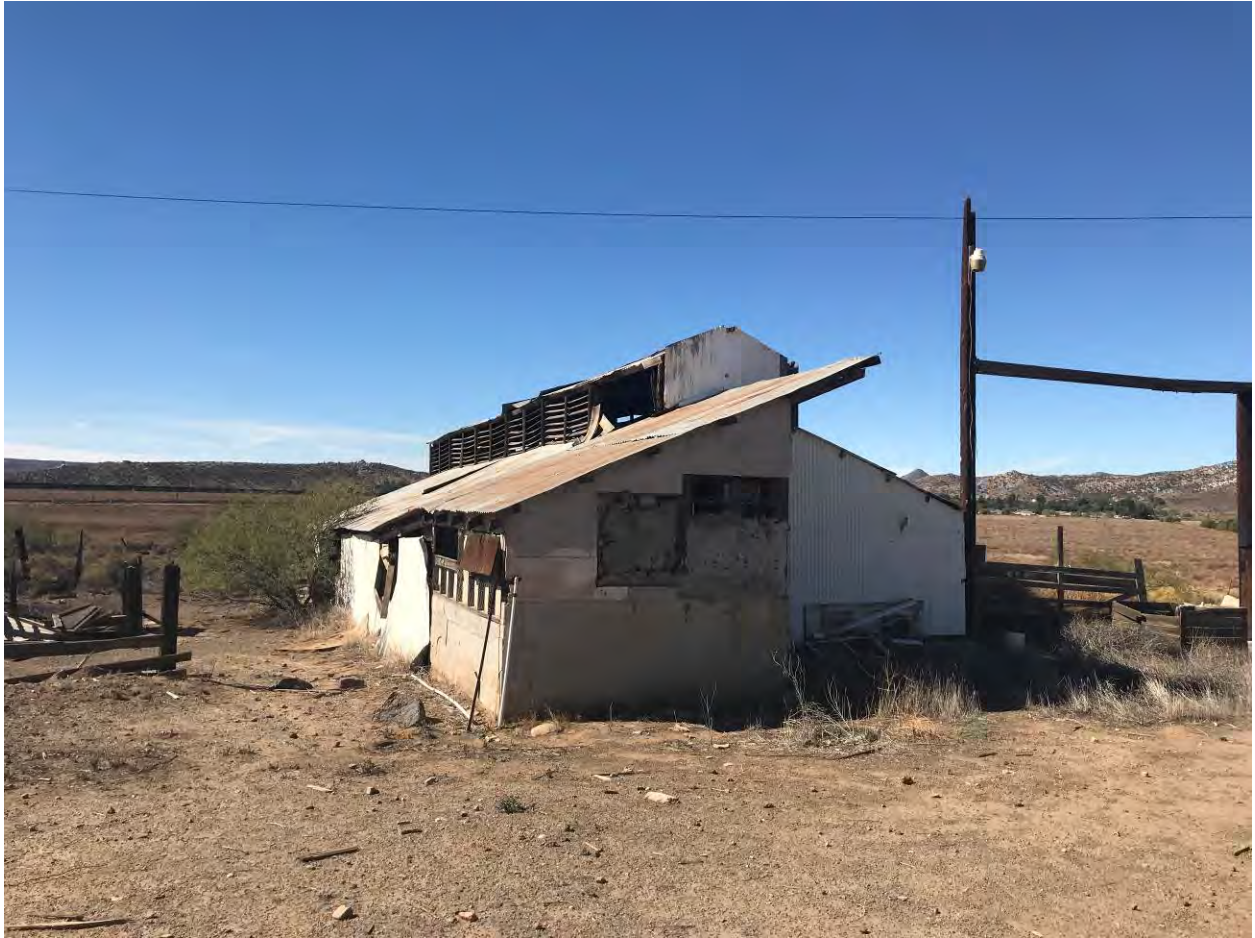
Photo 24 – Ground level view of the east side of Building 8.
