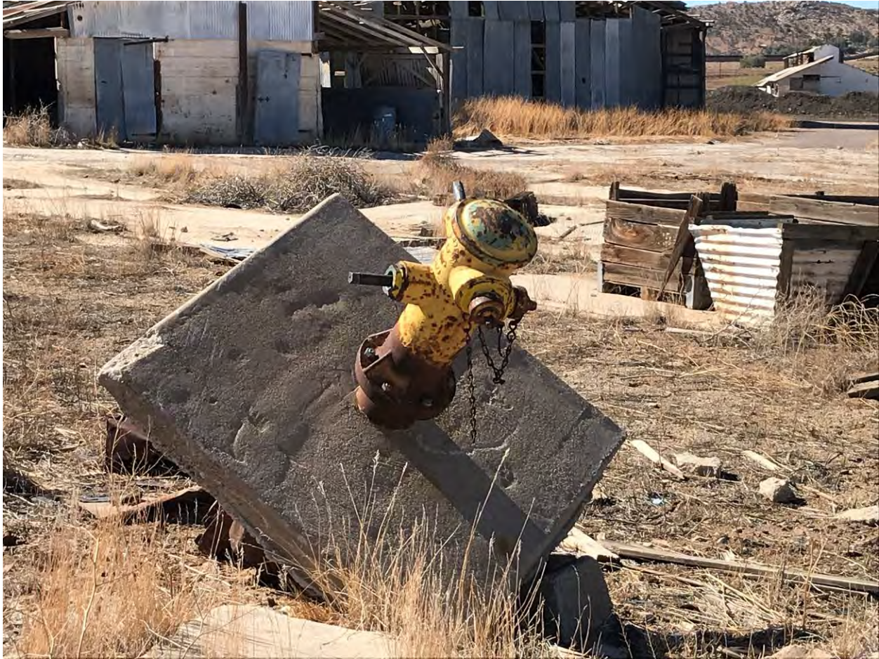
Photo 25 – Ground level view of the concrete pads north of Area 4. The fire hydrant was found to contain elevated lead levels.
