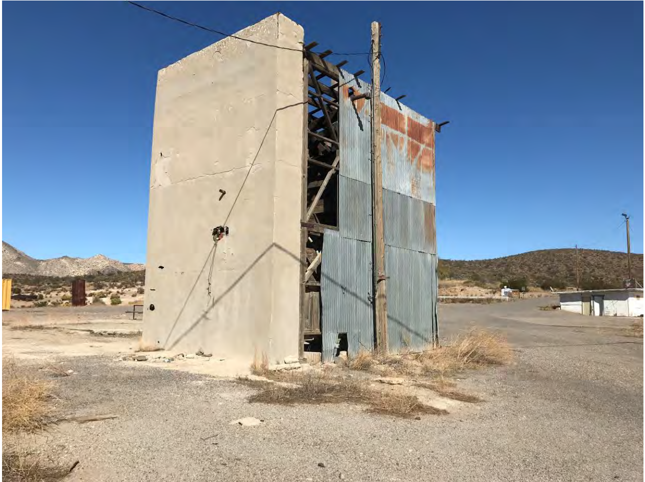
Photo 19 – Ground level view of the south and west sides of Building 4B.
