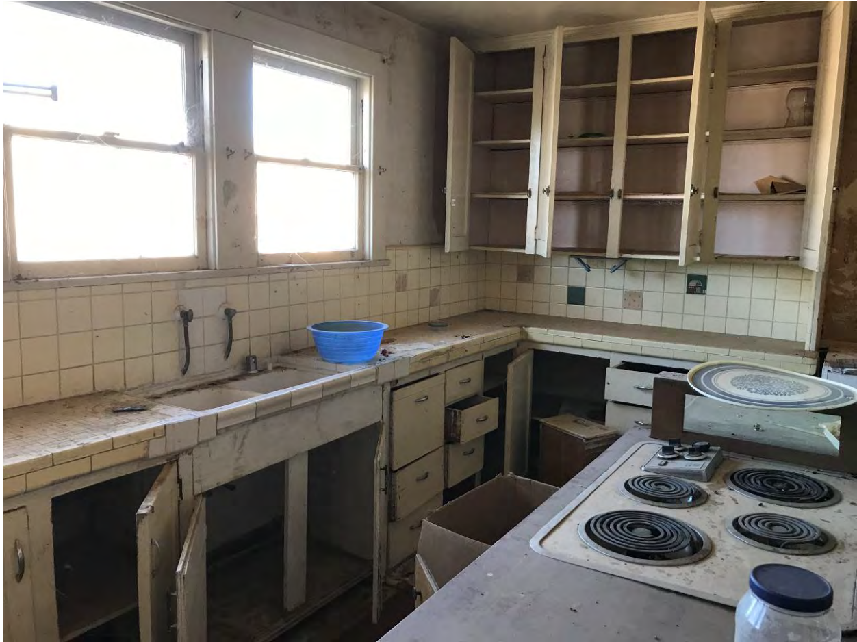
Photo Eight – Photo of ceramic wall tile and tile along the edge of the counter tops on sides A and B, and windows, window frames and window sills on side A of kitchen in building 6 that were found to contain elevated lead levels.
