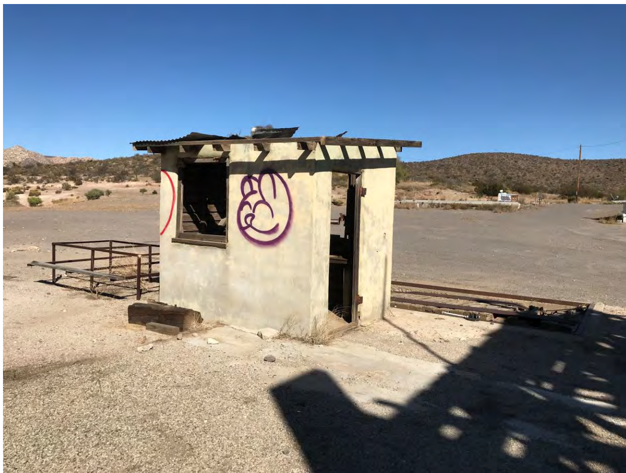
Photo 18 – Ground level view of the south and west sides of Building 4A.
