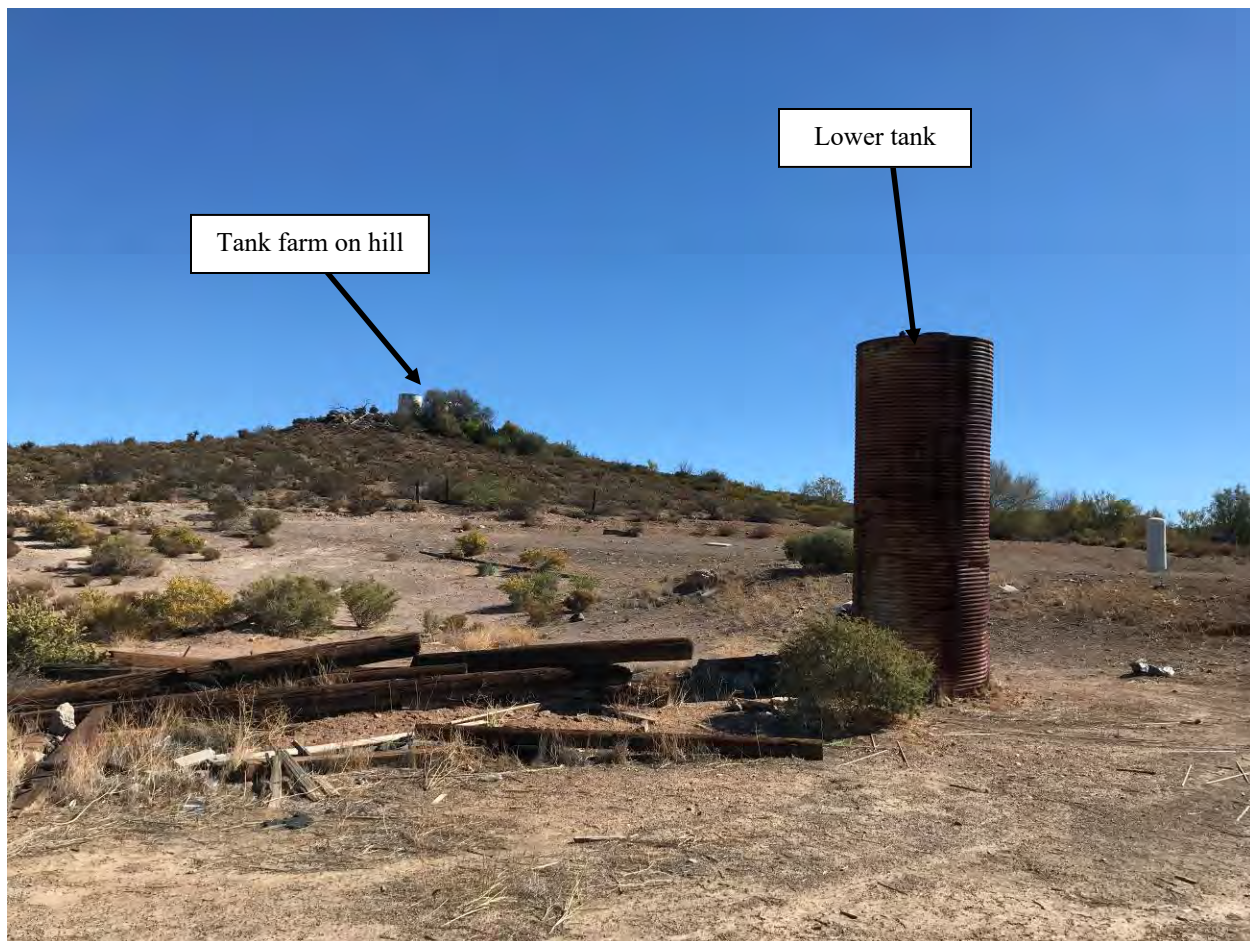
Photo 31 – Ground level photo of small lower tank below the tank farm on the hill northeast of the structures.
