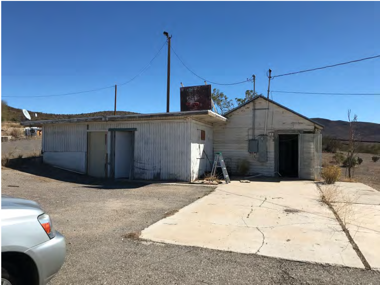
Photo Four – Ground level view of the west side of Building 5.
