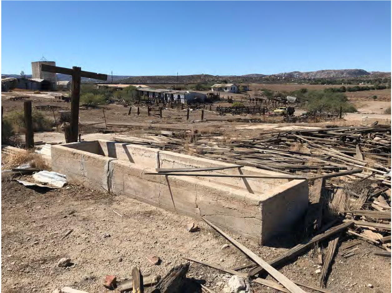
Photo 26 – Ground level view of the concrete pads and troughs at north end of the section of property with structures.
