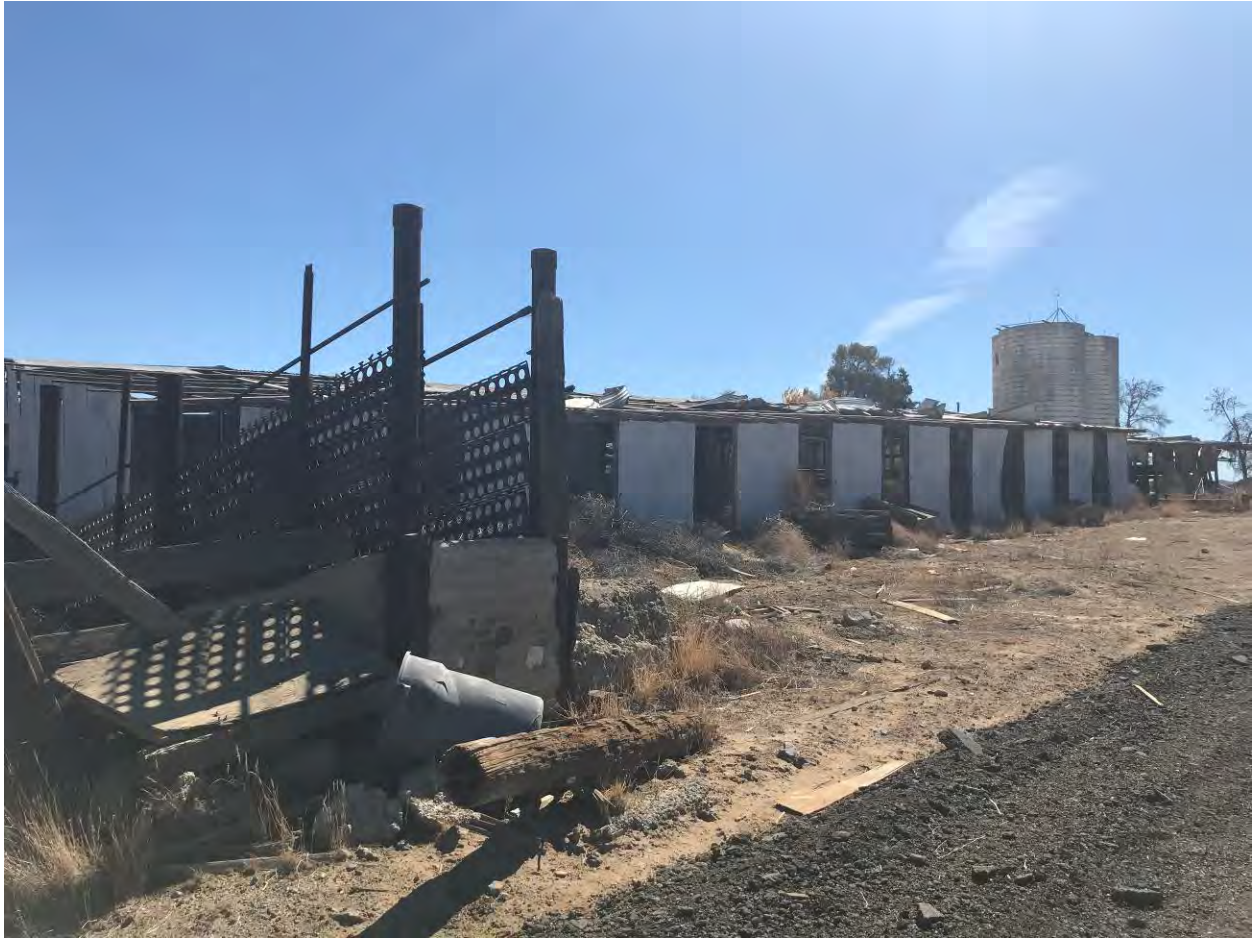
Photo 23 – Ground level view of the west side of Building 3.
