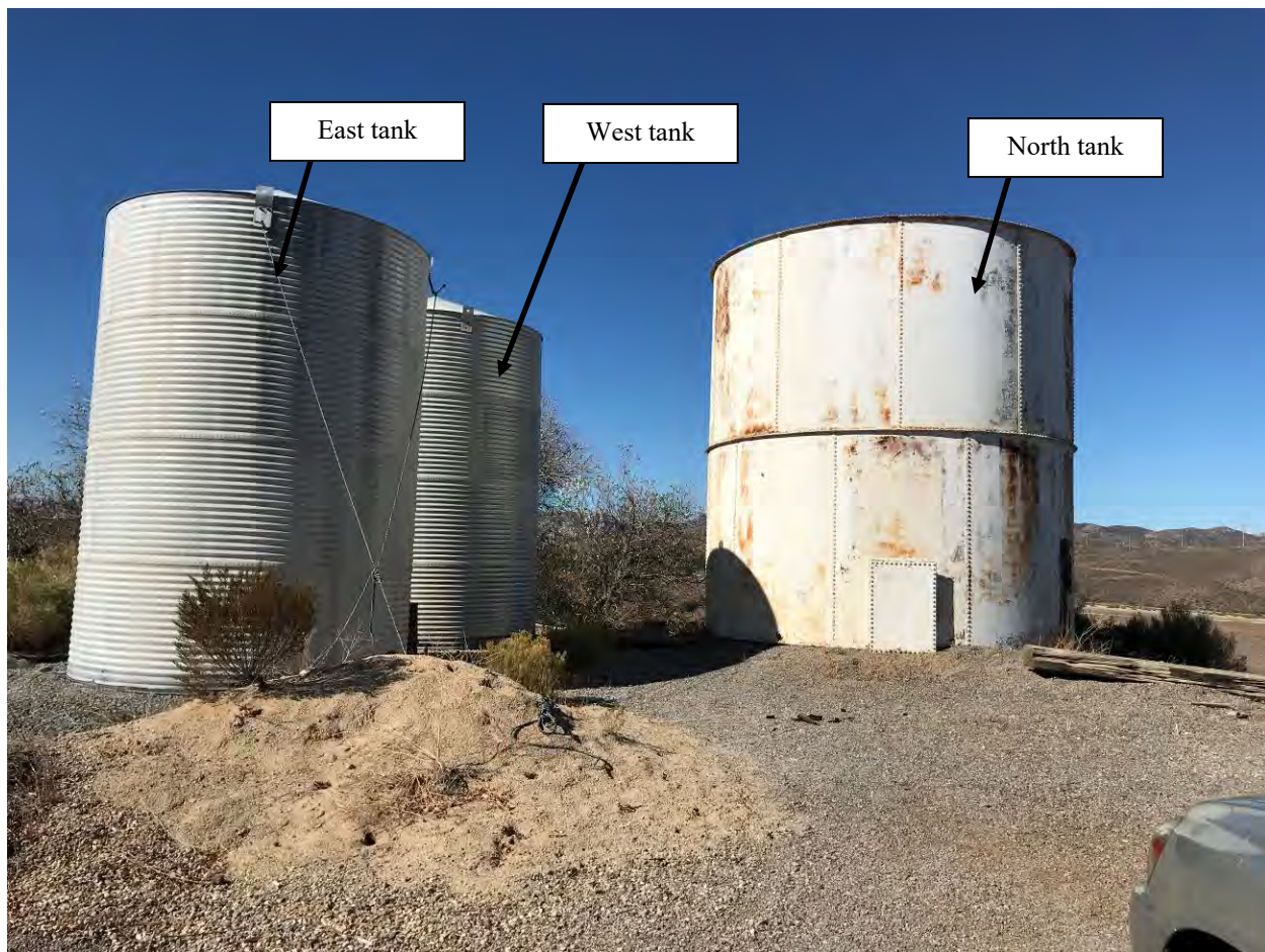
Photo 30 – Ground level photo of tank farm on the hill northeast of the structures.
