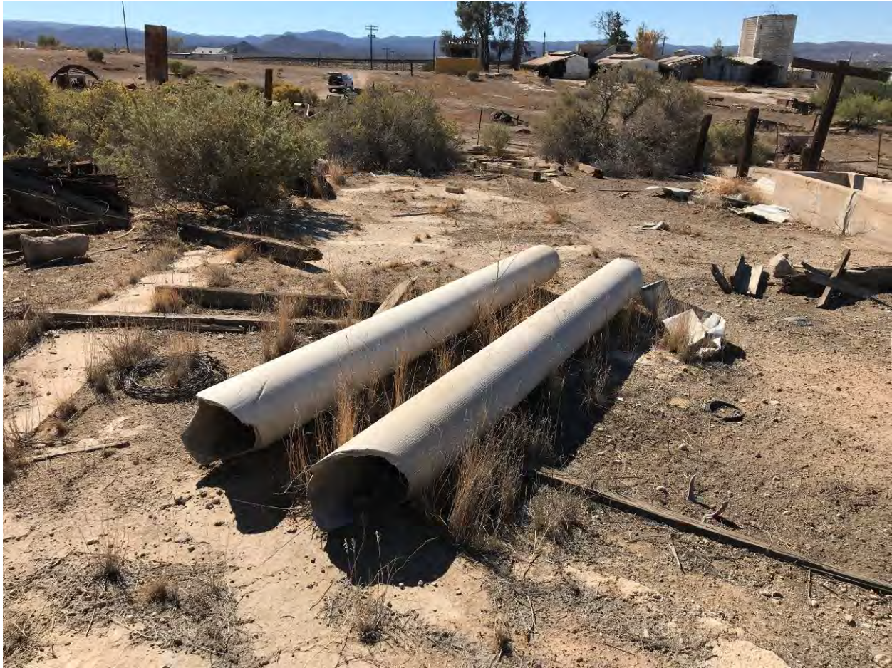
Photo 27 – The transite pipe located in several debris piles north of the structures were found to contain asbestos.
