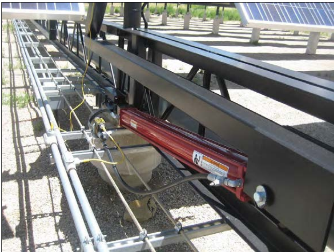
Figure 8: Example of a Tracking Solar PV Installation
