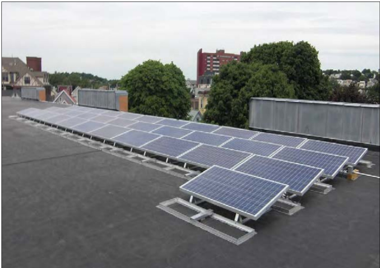
Figure 6: Example of a Roof-Mounted Solar PV System
