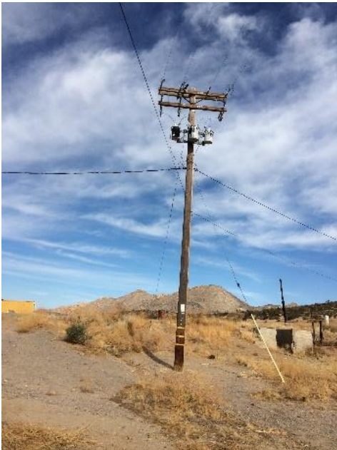
Photograph 23 – Three pole-mounted transformers located on the ranch.
