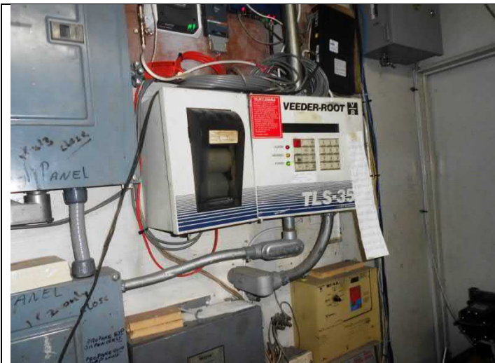
11. Continuous automatic monitoring system (Veeder Root)
