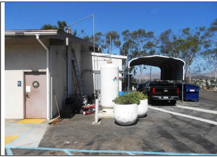
13. View of vapor recovery unit and vent pipes
