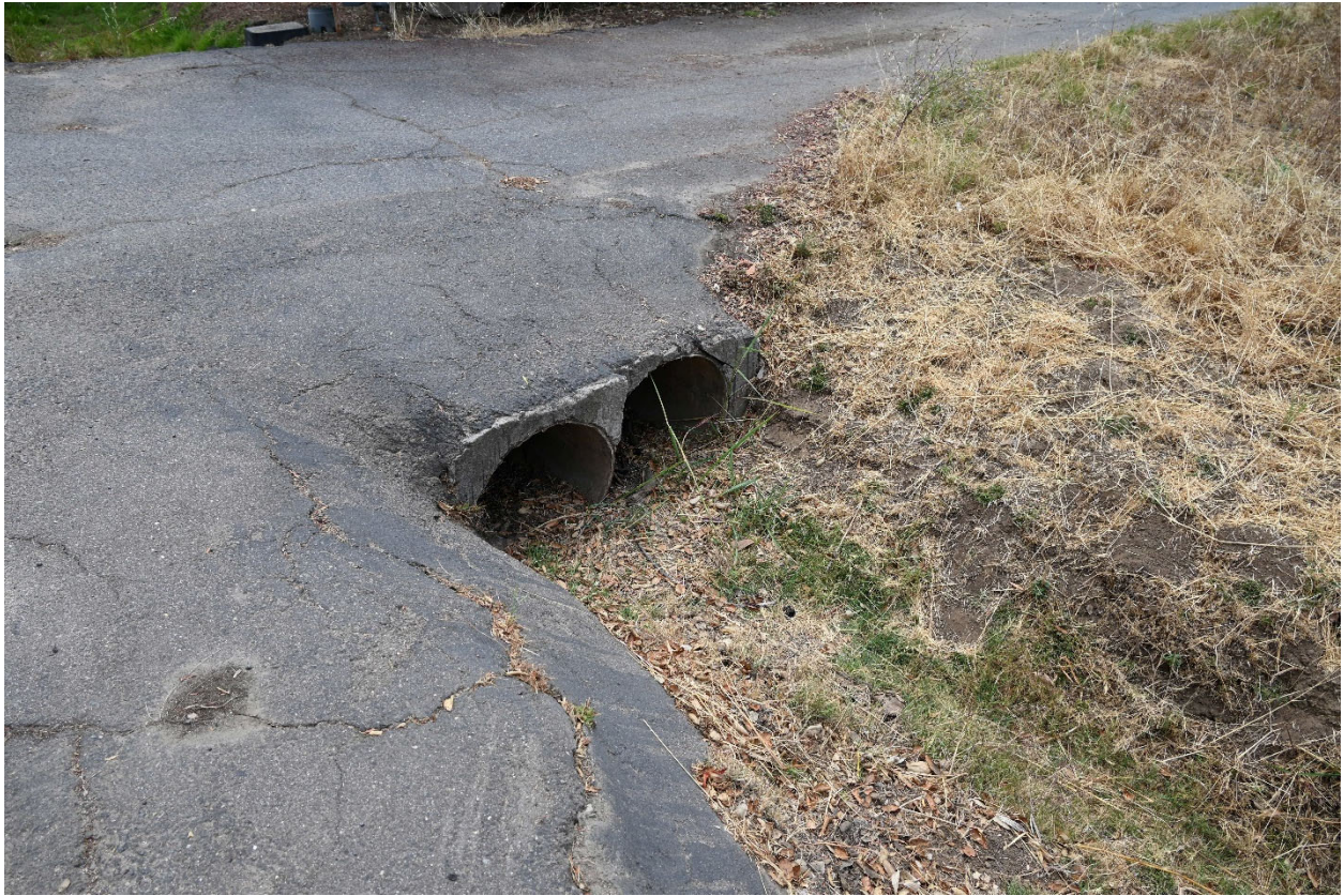
Figure 11. Second Grade Control at Downstream End of Reach 2
