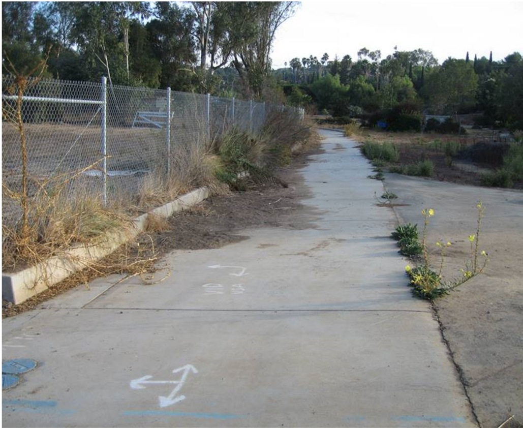
Figure 1. Concrete Swale that Collects Project Runoff (project is left of fence)
