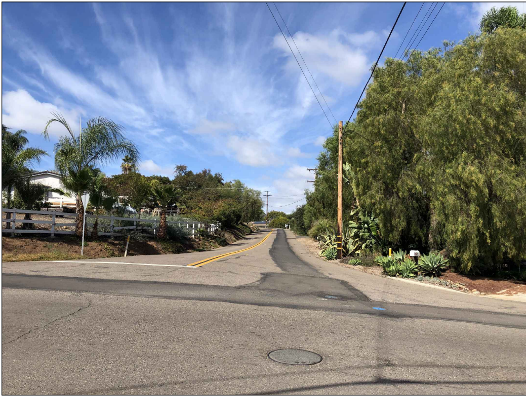
NEAR POINT B LOOKING TOWARDS MONTGOMERY DRIVE
