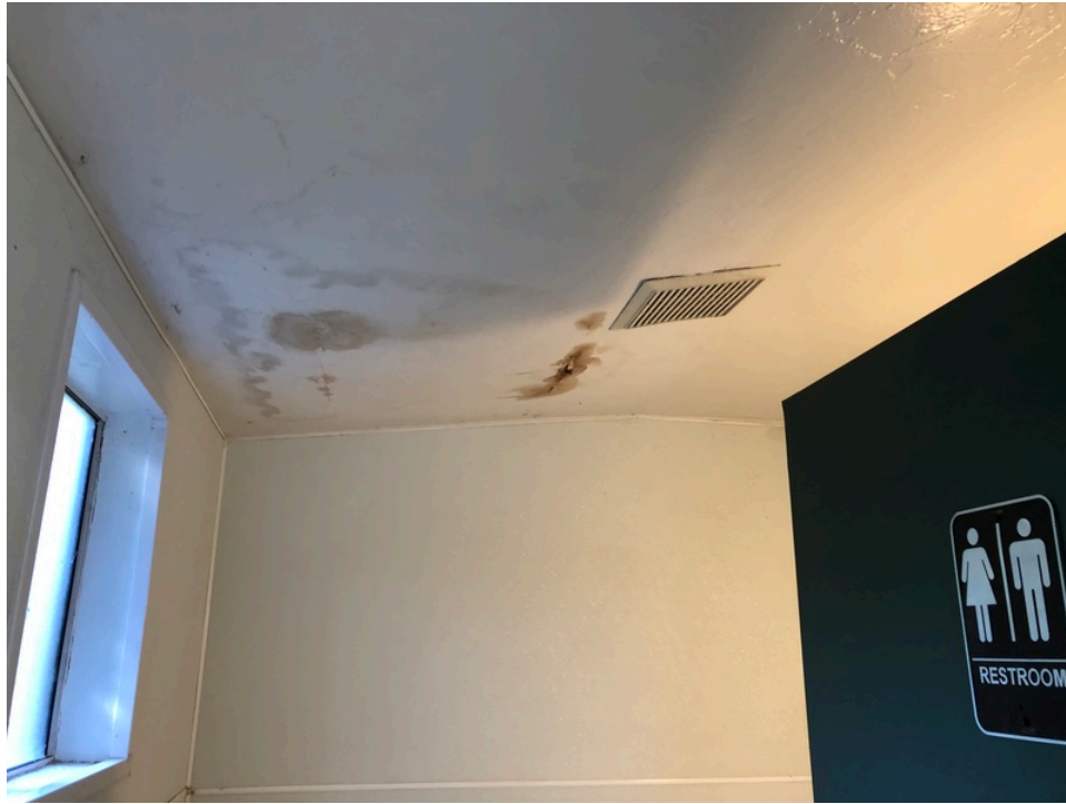
17. Past moisture intrusion observed in the restroom
