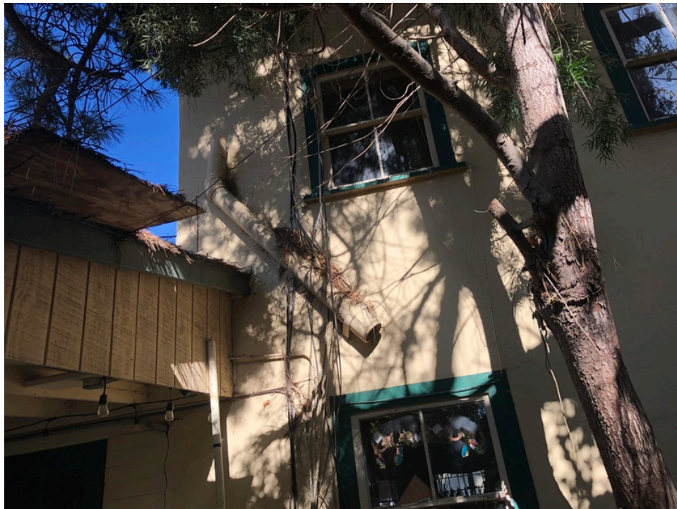
18. Suspect ACM piping on the south elevation of the retail candle store
