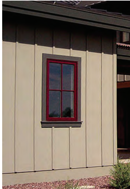
1 VERTICAL SIDING BY: HARDIE PANEL
