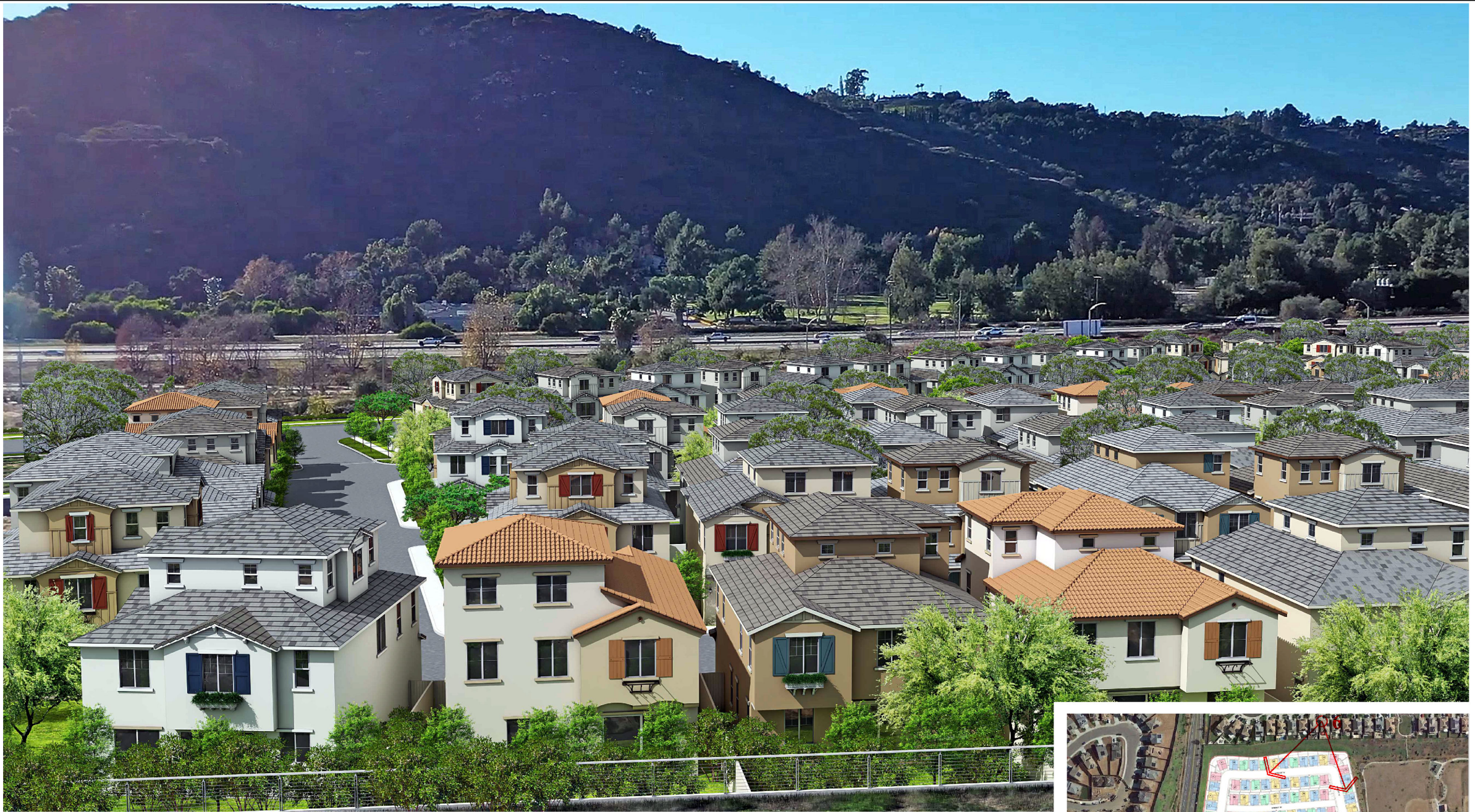
SITE OVERVIEW @ SOUTH PARCEL
