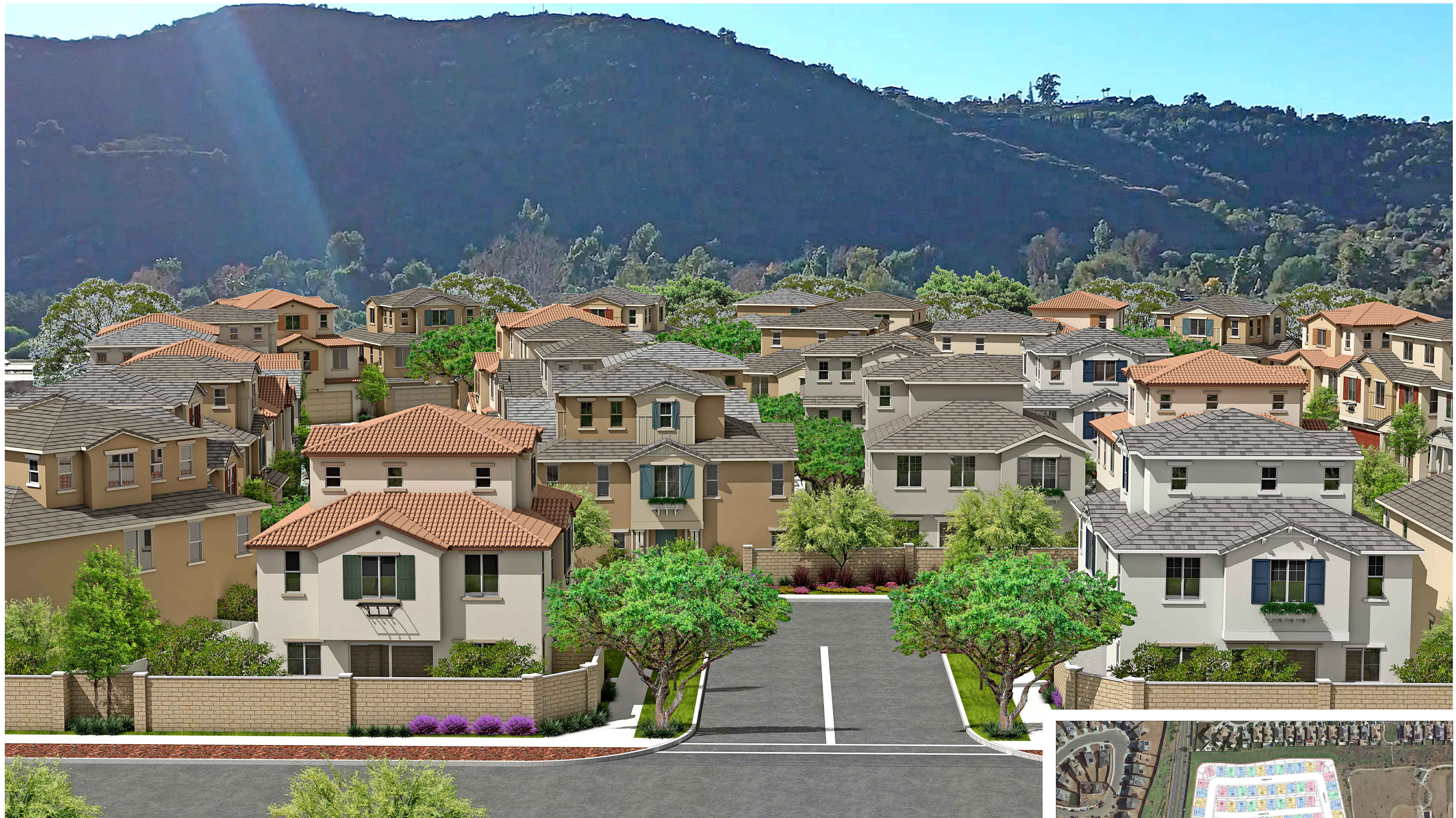
OVERVIEW @ NORTH PARCEL
