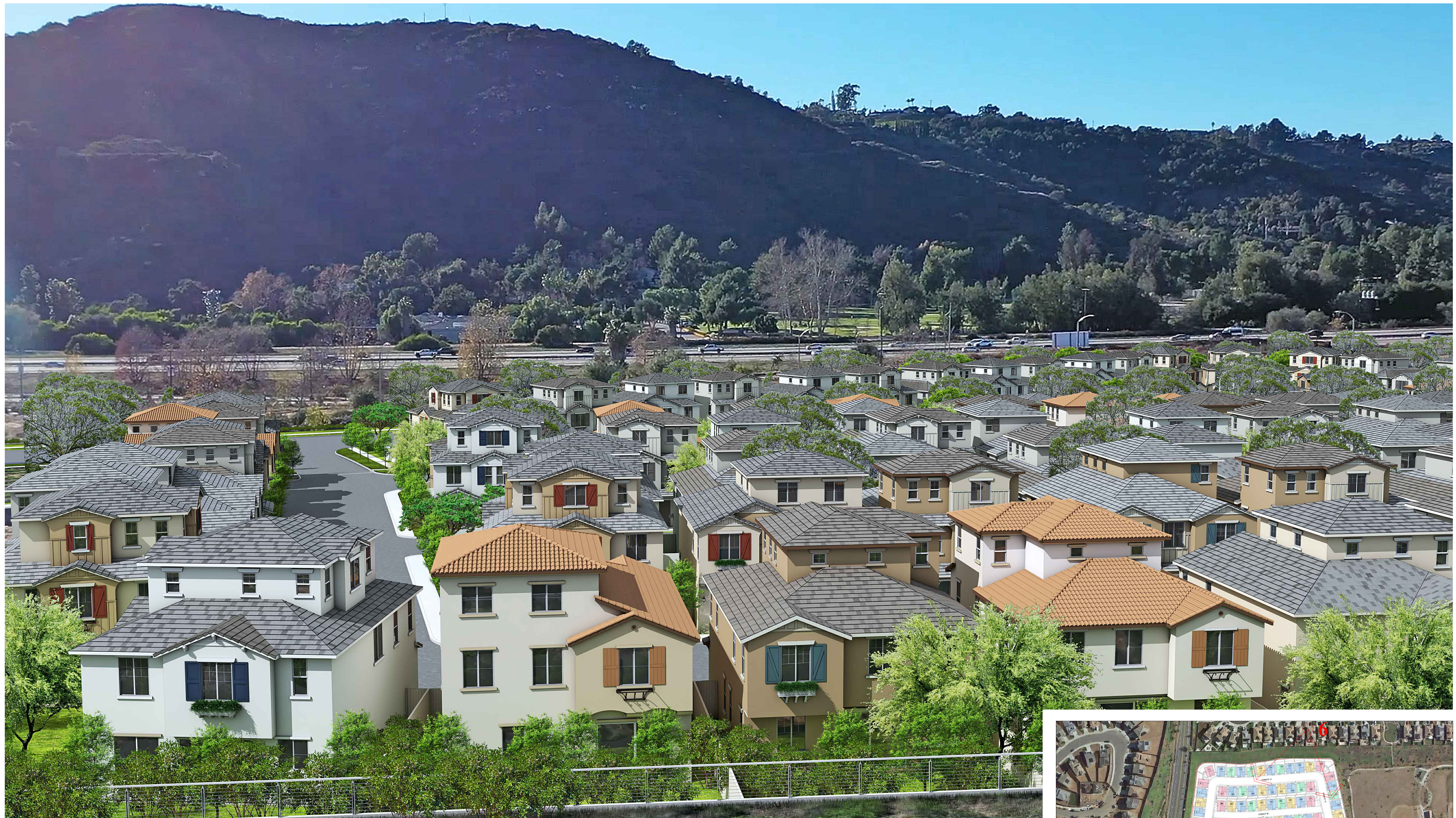
SITE OVERVIEW @ SOUTH PARCEL
