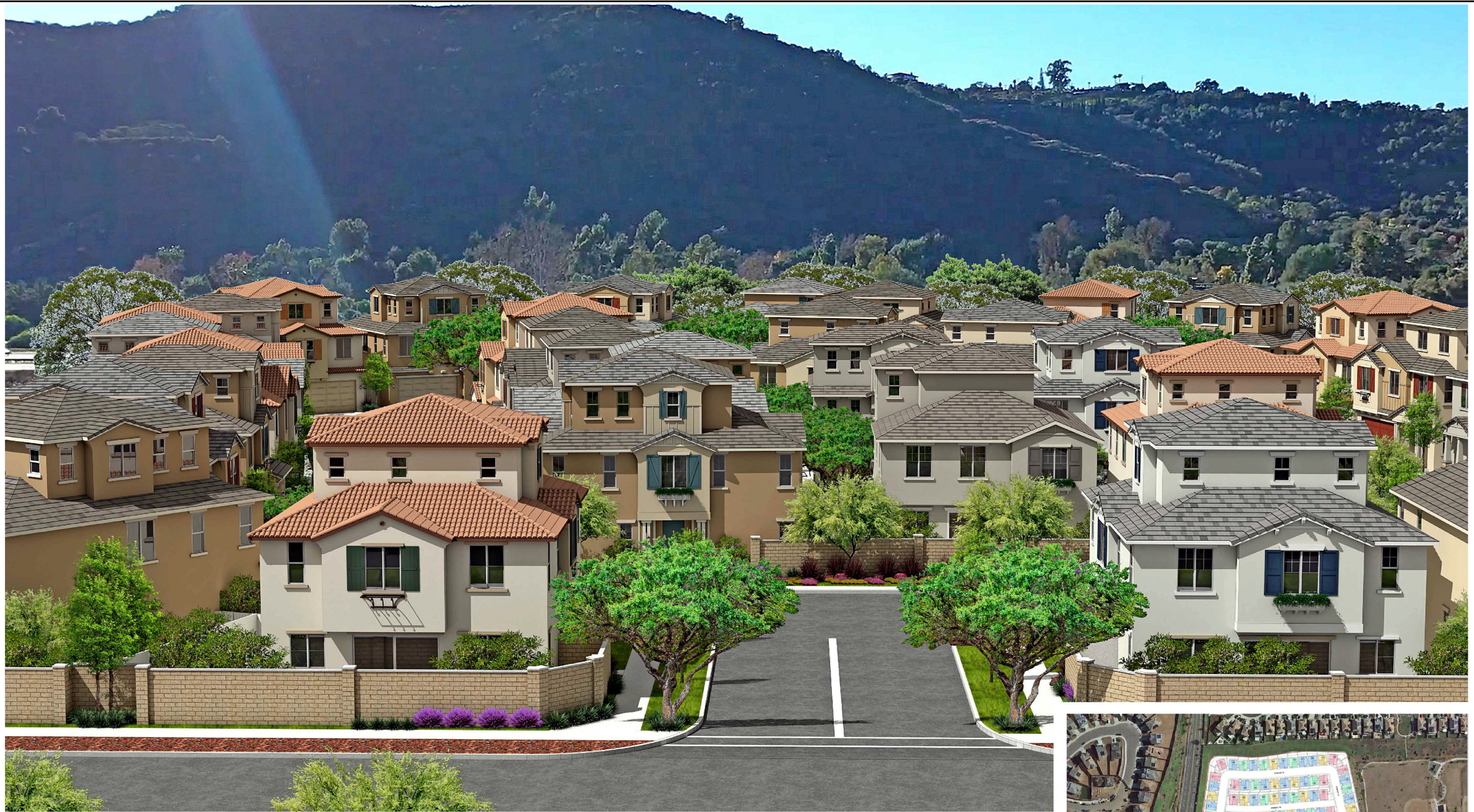
OVERVIEW @ NORTH PARCEL
