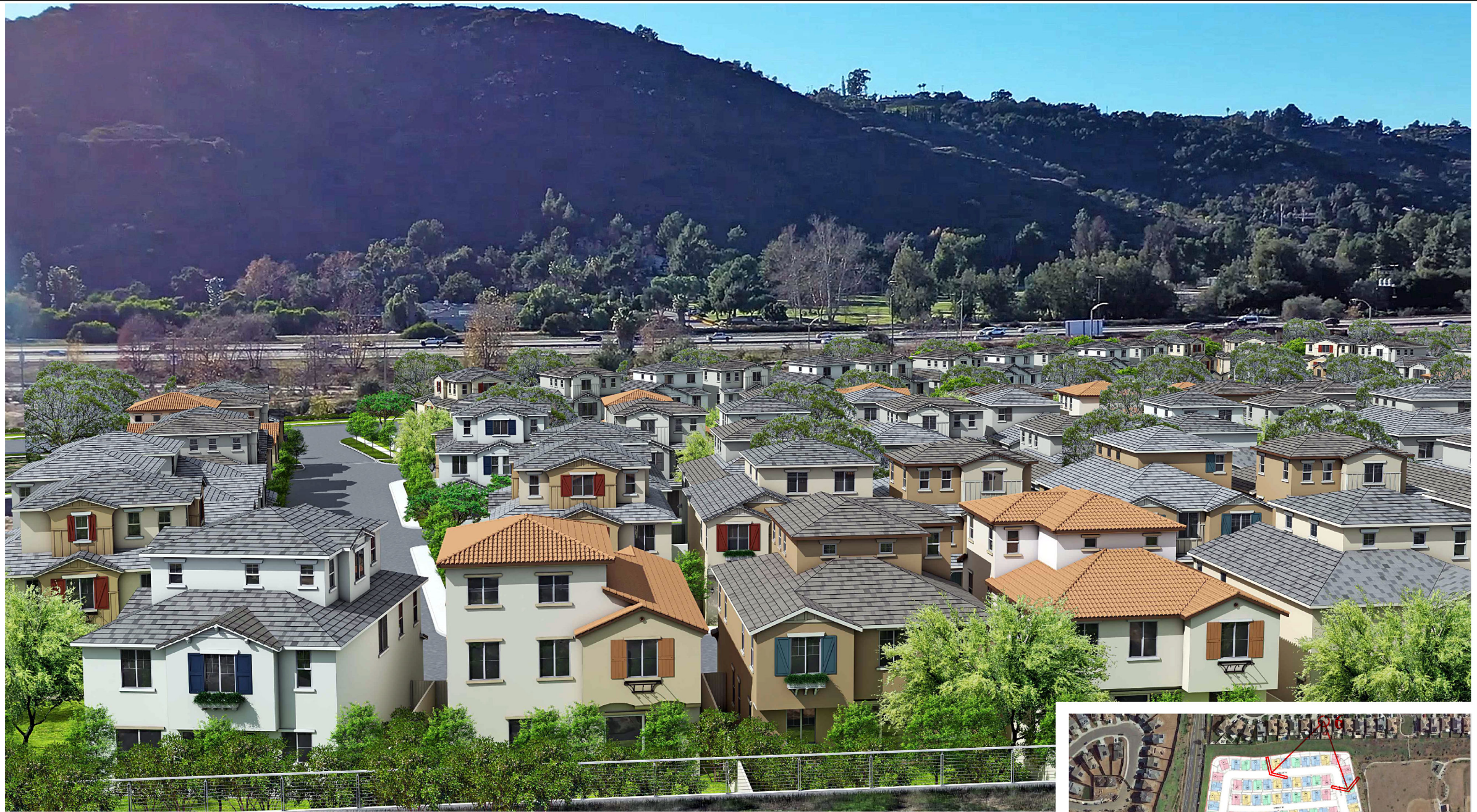
SITE OVERVIEW @ SOUTH PARCEL
