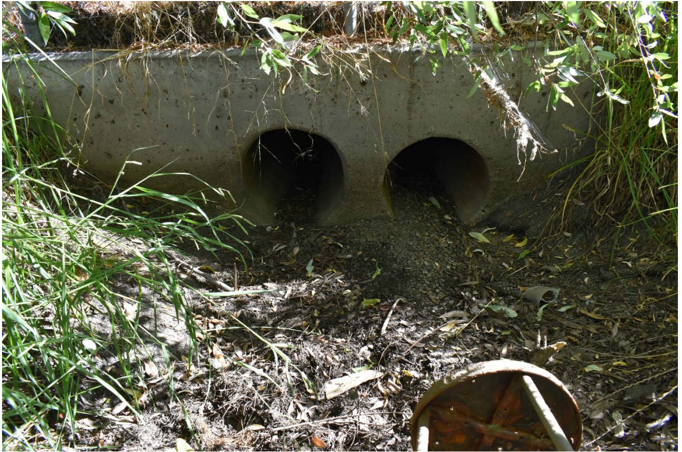
Figure 1. Double 18-inch RCP Outlets at Upper End of Reach 1
